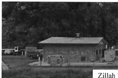
Zillah Wastewater Treatment Plant
