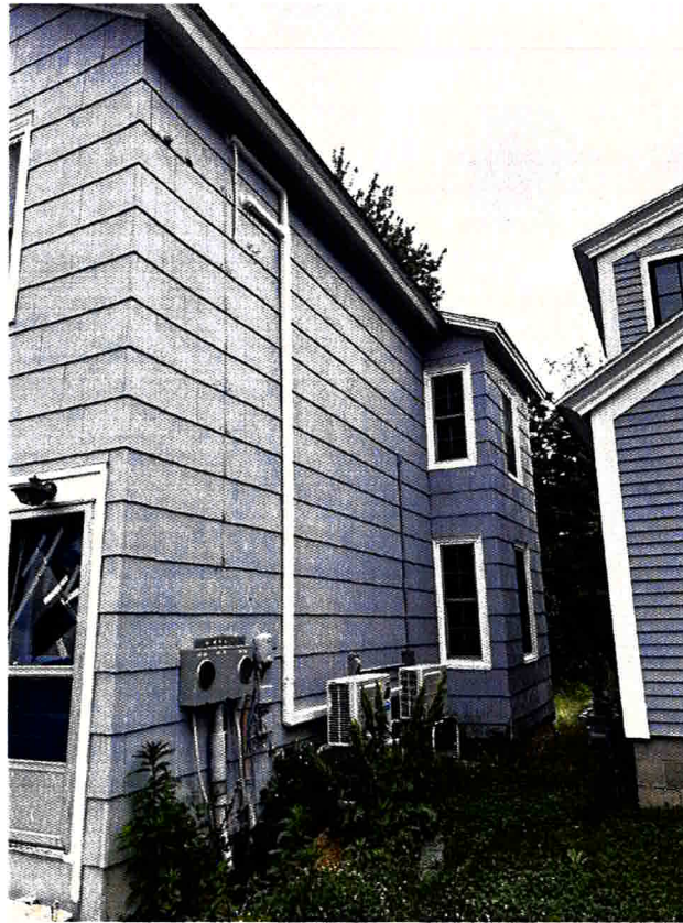
SOUTHWEST FACING SIDE – ALONG ELY / MELCHERT PROPERTY LINE
