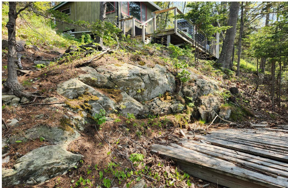
Bedrock Supporting Existing Building
