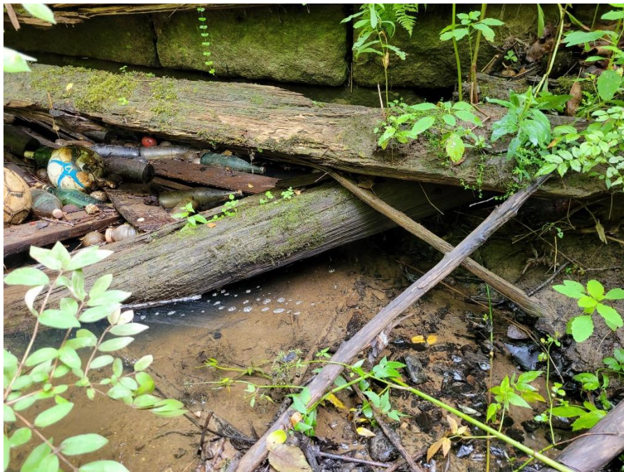
View of stone culvert inlet looking easterly.
