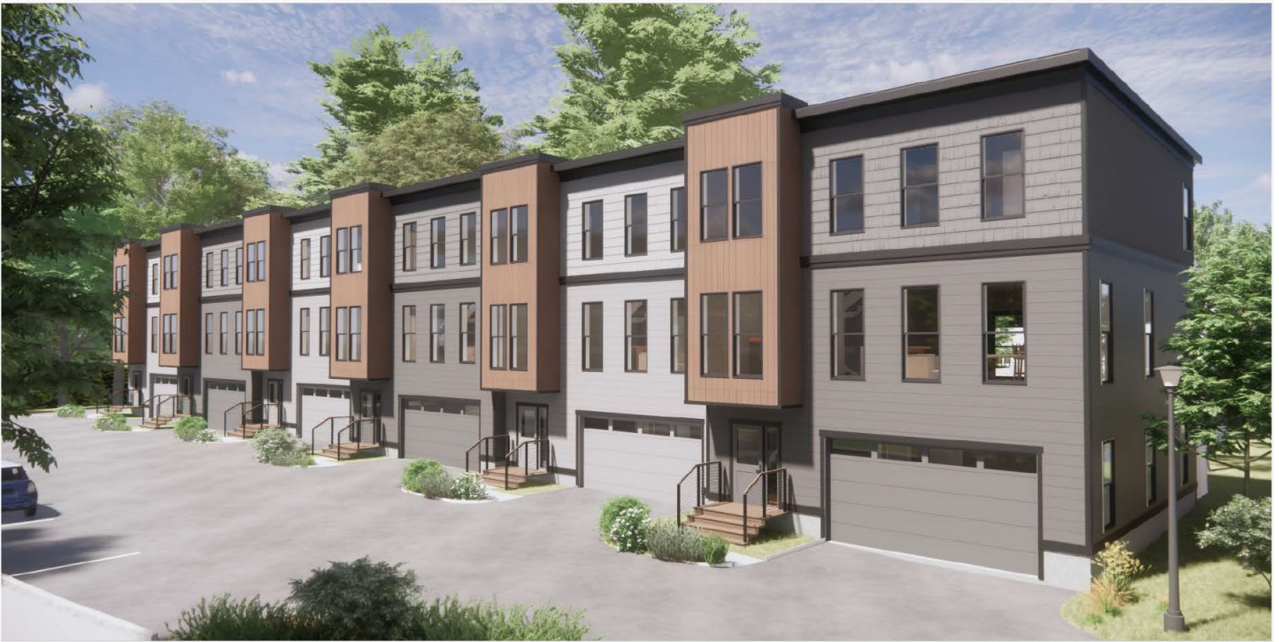
Townhomes (Building 4): Internal Railroad Square Elevation
