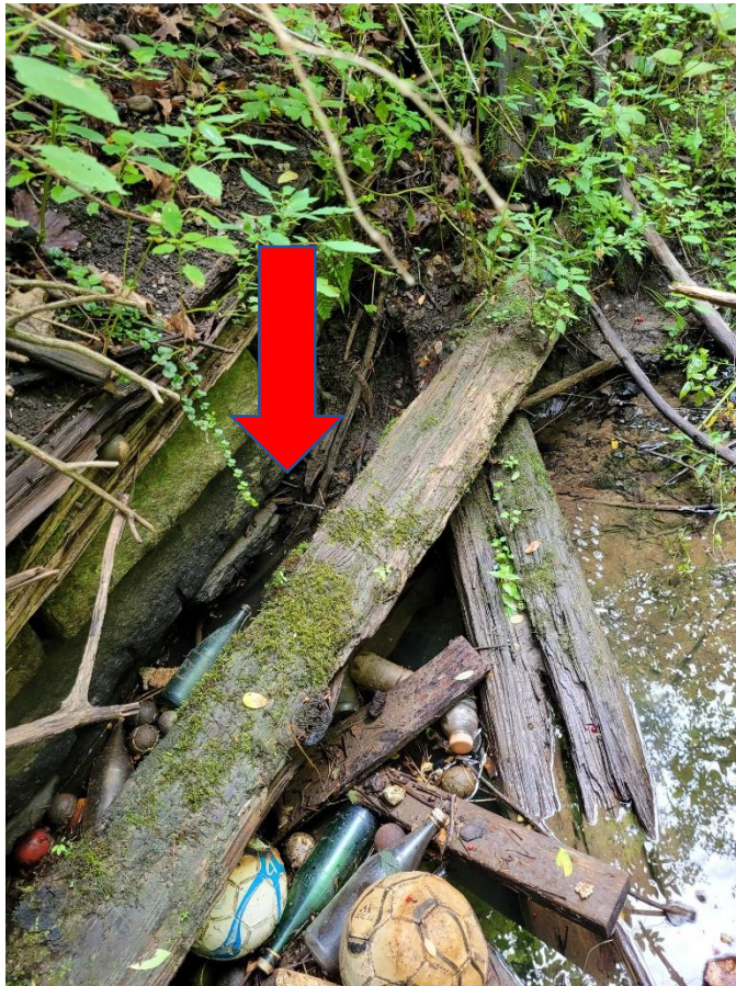
View of stone culvert inlet looking southerly. Note crown of culvert.
