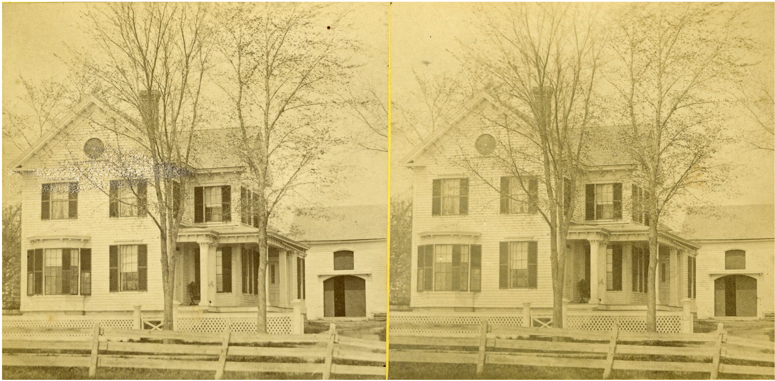
This one likely dates to around the turn of the 20 th century We have some sources that suggest that the bay window was installed between 1903 and 1911.
