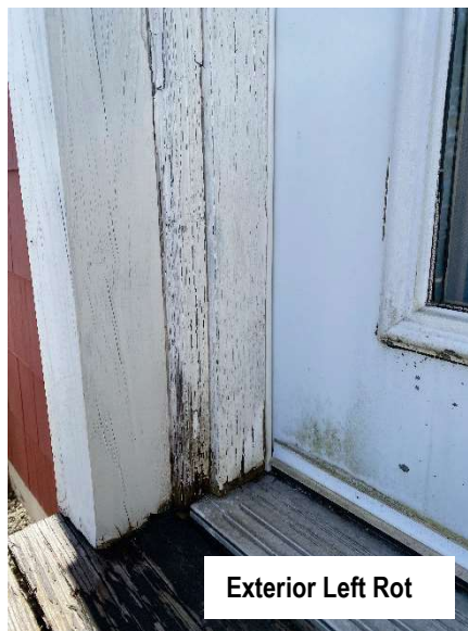
Figure 7. Images of French Door Rot and Interior Damage
