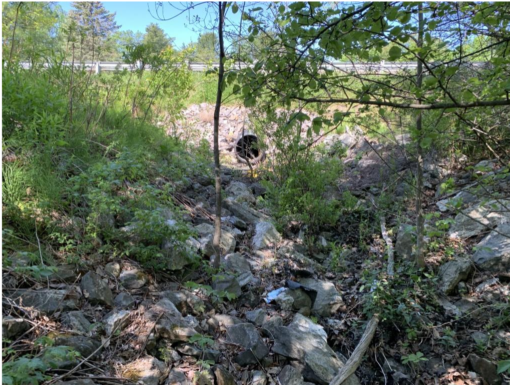
Stormwater outfall to upland drainage ditch from Route 1.
