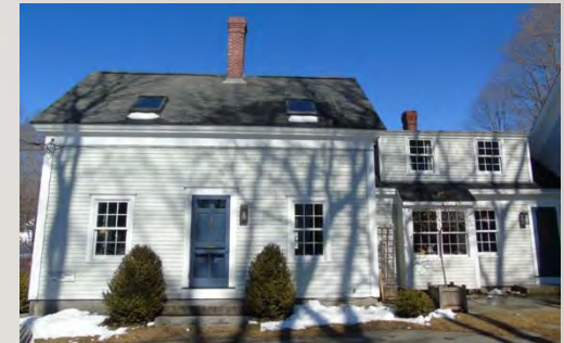
Patrick Haney House c. 1849, 58 Hillside Street
