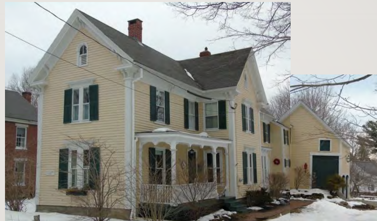
Charles W. Jordan House & Barn 1877, 42 Center Street
