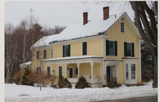
Harvey House, 1859, 109 Main St.
