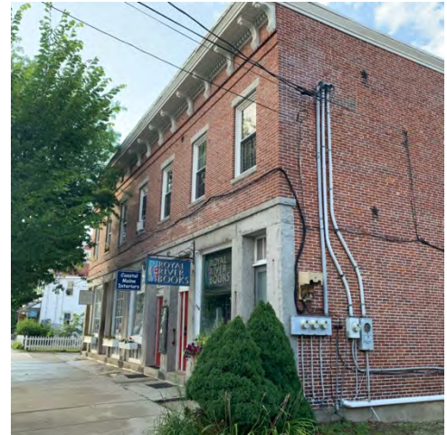
The Brick Block, 355, 357, 359 Main Street.
