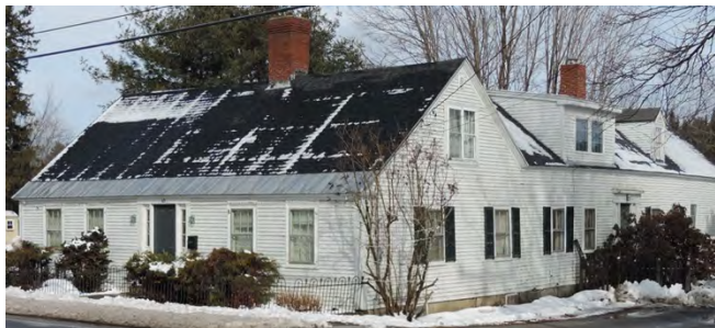
Matthias Storer House, 43 West Main Street.
