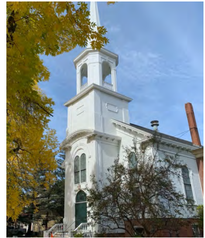
The Italianate style Central Parish Church (now First Universalist), 97 Main Street, is a focal point of the Lower Village designed by architect Augustus Holt.
