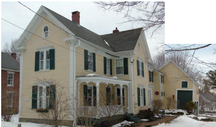
Charles W. Jordan House & Barn, 42 Center Street.
