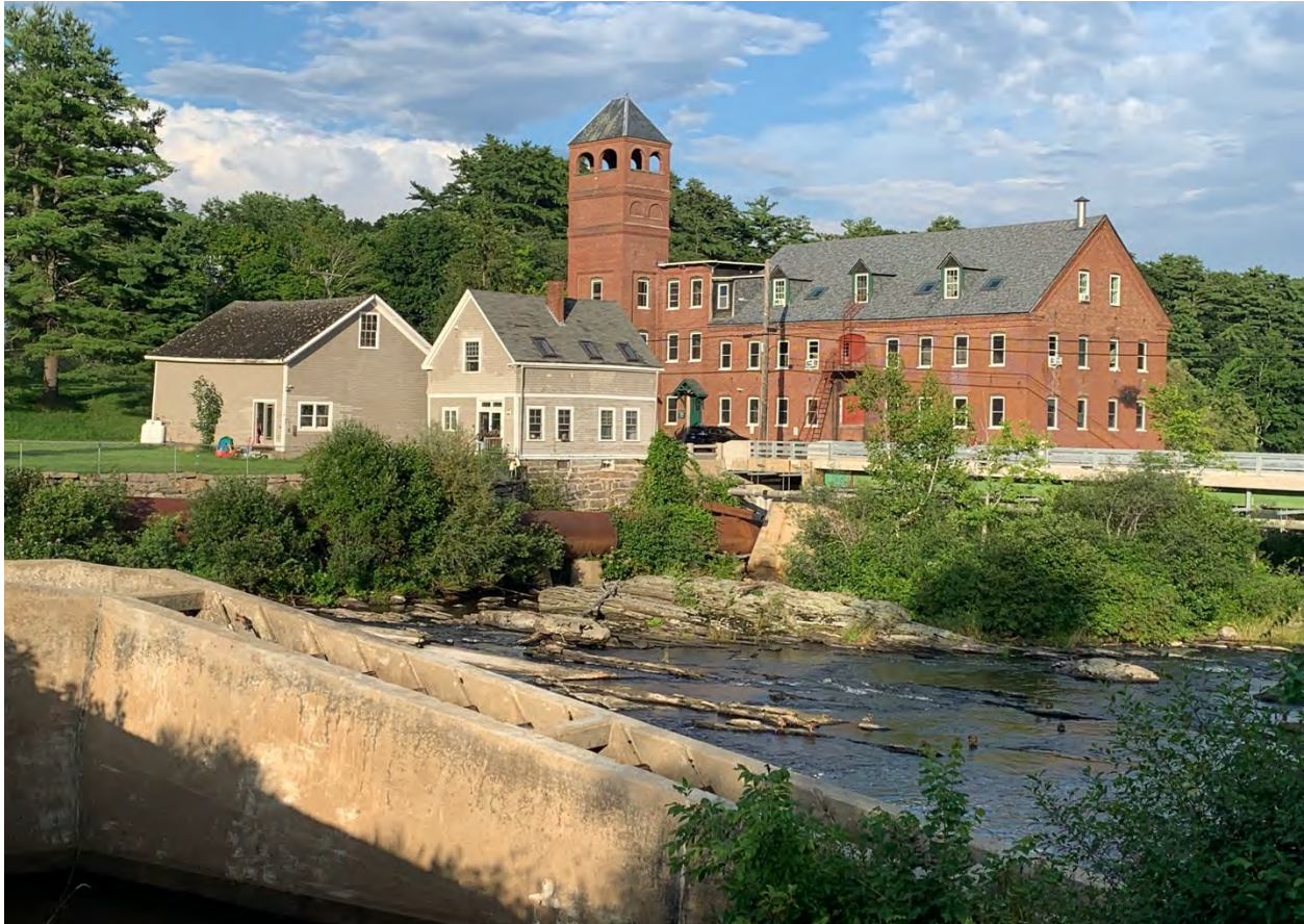
The brick Royal River Manufacturing Company complex, now known as the Sparhawk Mill, at 81 Bridge Street, with the former company office and barn across the street at 80 Bridge. Architect Francis Fassett designed the office and the Italianate tower. Photo: H. Bassett.
