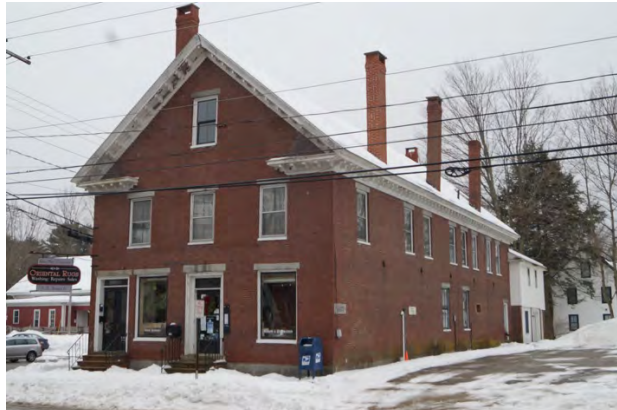
Storer General Store, 108 Main Street.
