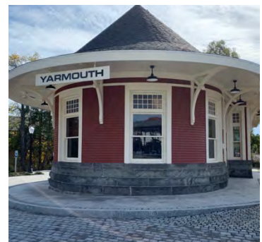
Grand Trunk Depot, 288 Main Street.
