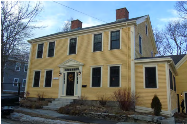
Ebenezer Corliss House, 9 Church Street.
