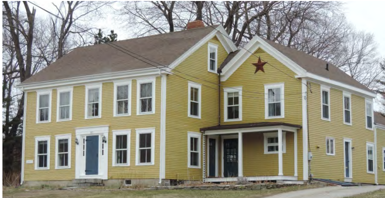
John Cutter House & Barn, 163 West Main Street.
