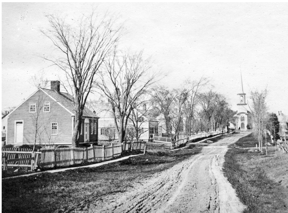
An early view of the Lower Village looking up Portland Street toward Main Street with the former Central Parish (now Unitarian Universalist) Church as a focal point, c. 1875, Photo: Yarmouth History Center.
