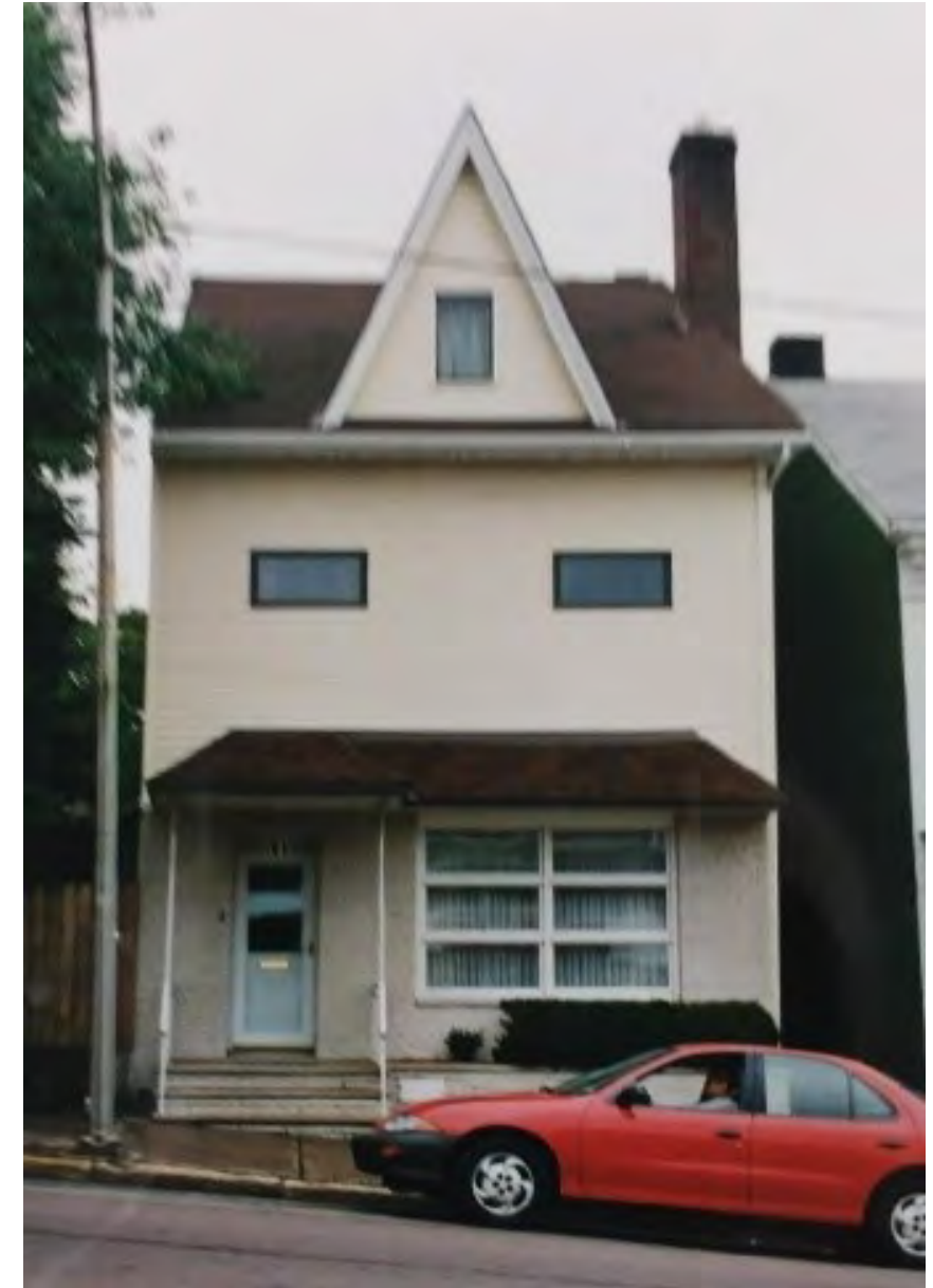
An example of how window infill and modern window replacements can dramatically change the visual character of a building.
