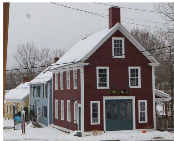
Fire Station, 50 Main Street.
