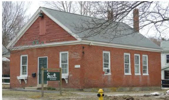
School, District No. 4, 117 West Main Street.
