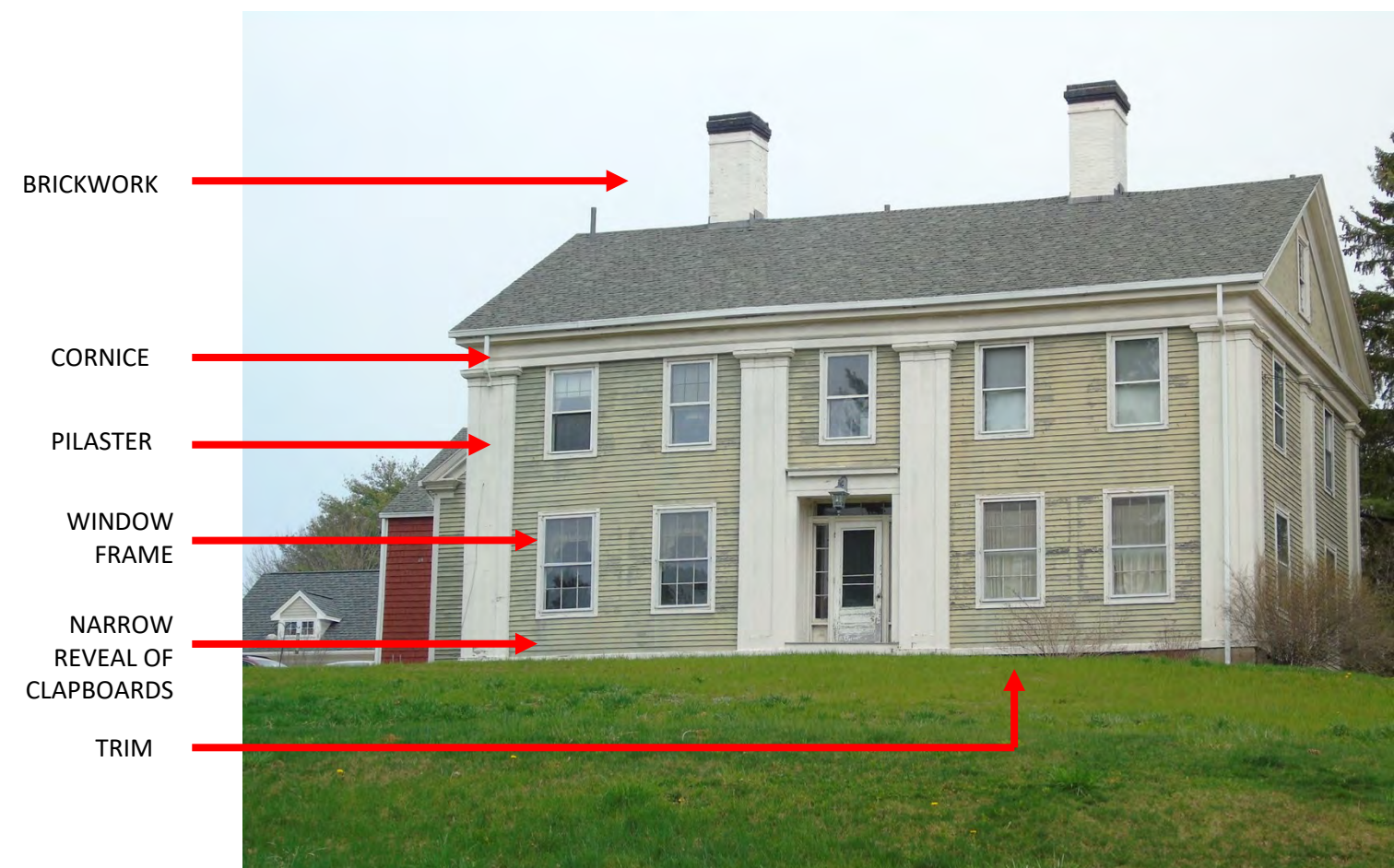
Without the architectural details (including window frames, pilaster, window frames, cornice, and decorative brickwork) this building would not have as much visual richness or sense of history.
