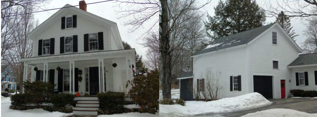
Edward H. Smith House & Barn, 65 Center Street.
