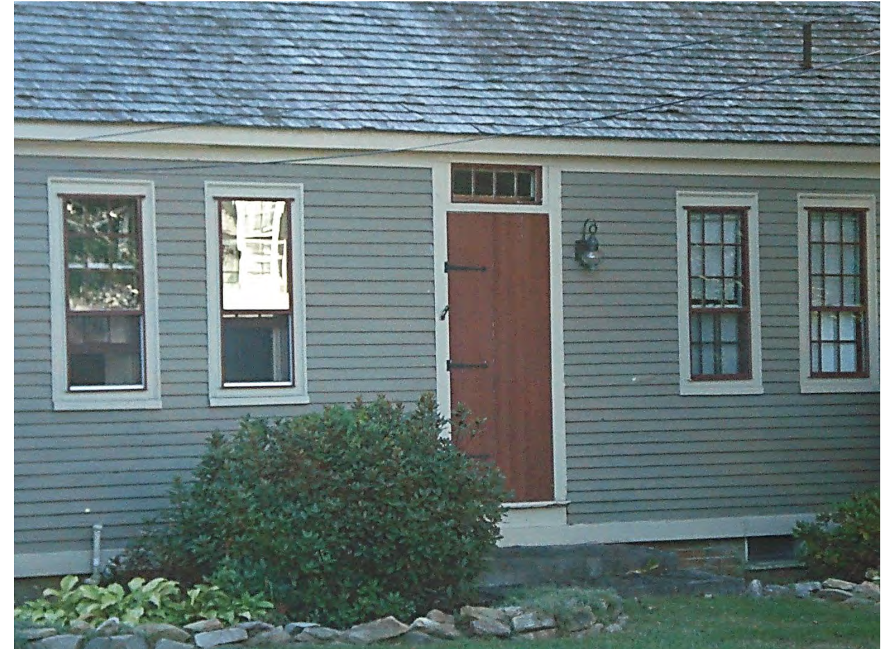
A board and batten storm door on this Yarmouth house provides distinctive character to the building, and continues to function after decades/
