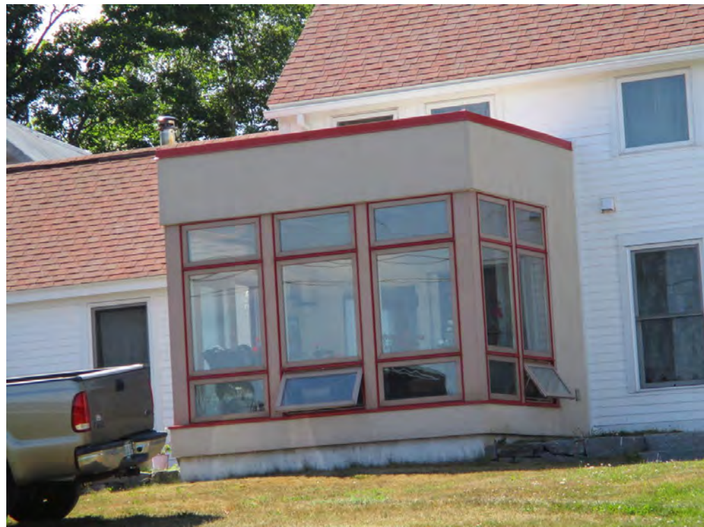
This addition makes no effort to respond to the materials or character of the original structure.
