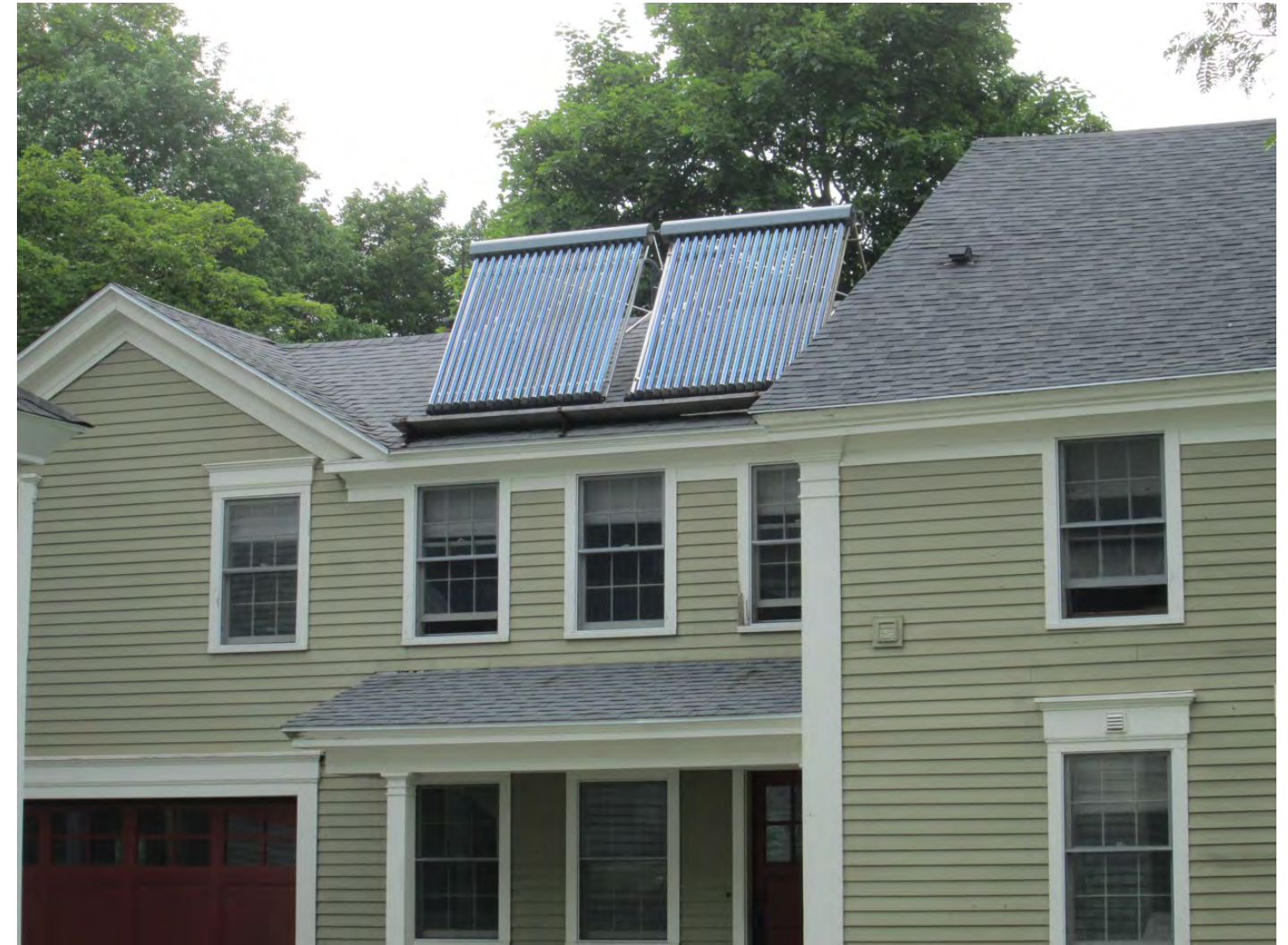
Avoid this scenario: device mounted at a high-profile angle on street facing facade.
