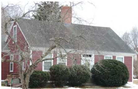
Alexander Mills House, 54 West Main Street.
