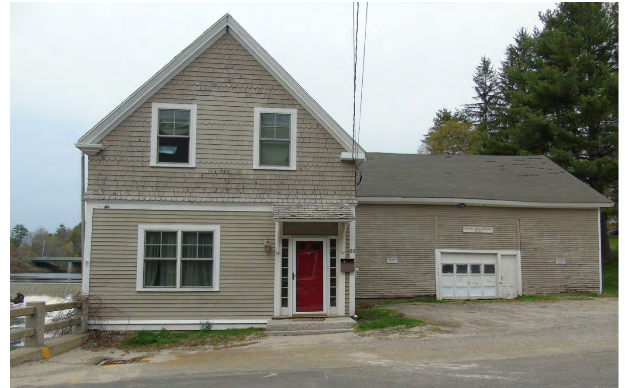
The decorative shingle siding of this 1880 house illustrates the rich texture of historic fabric.
