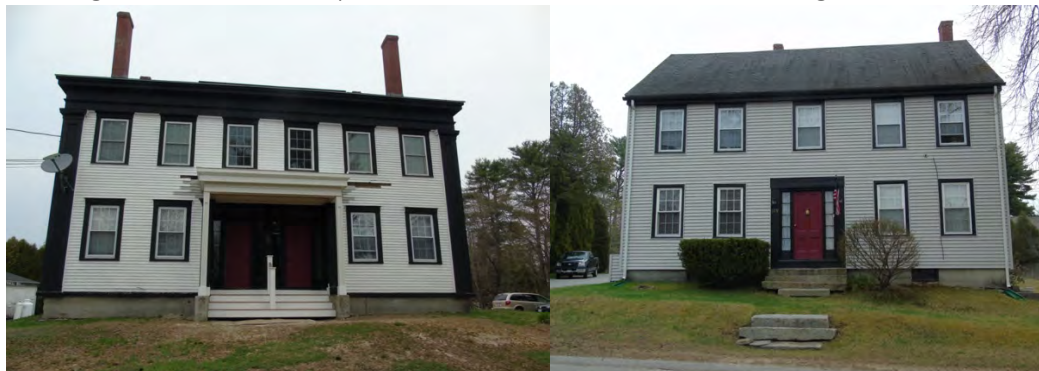
Worker housing for the Royal River Manufacturing Company at 107 and 109 Bridge Street (right).
