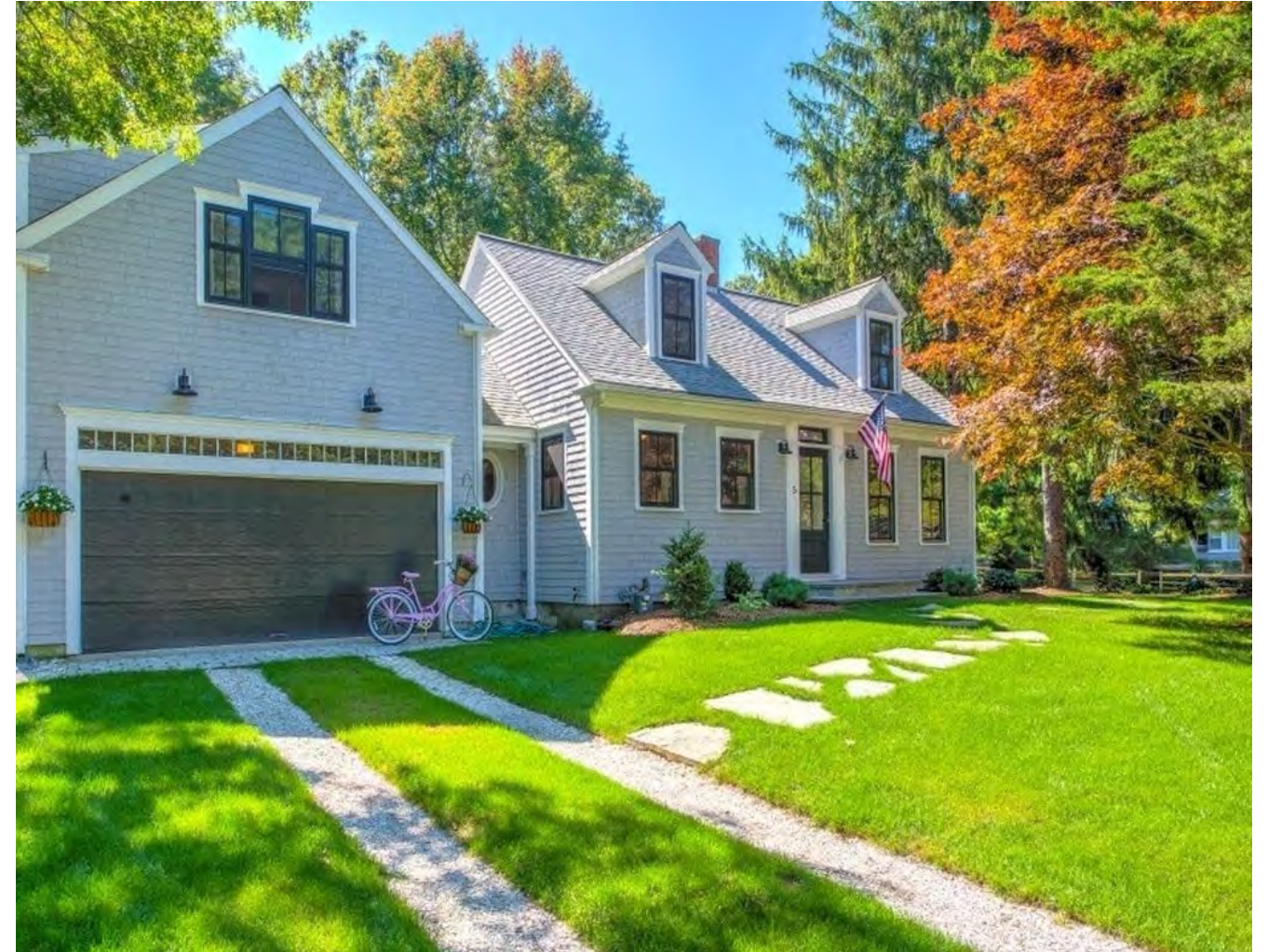
The garage addition is improperly scaled, and overwhelms the original structure.
