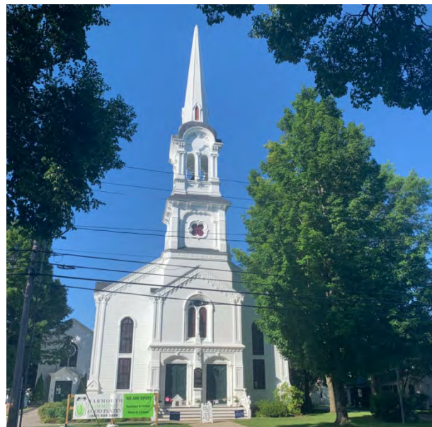
First Parish Congregational Church, 116 Main Street, Photo: H. Bassett.
