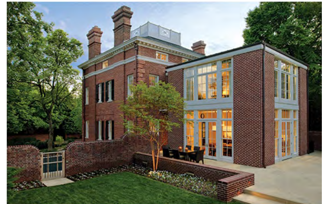
Materials in this addition are compatible in type, rhythm, texture, scale, and color with the original and surrounding buildings.
