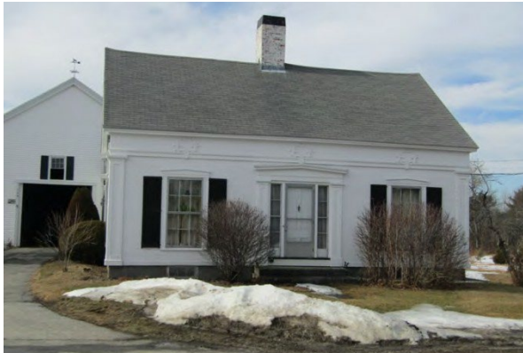
The cape at 159 Portland Street is a fine example of a gable ended, center hall Greek Revival style house, which retains its original details and attached barn and illustrates the rural character of the Town beyond the Village center.
