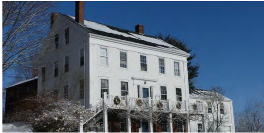
The Jeremiah Baker House, 35 East Main Street, was built c. 1848, with a brick basement that was used as a store. It is visible at upper right in the photo below.
