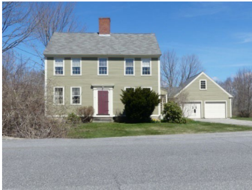
Allen Drinkwater House, 310 Gilman
