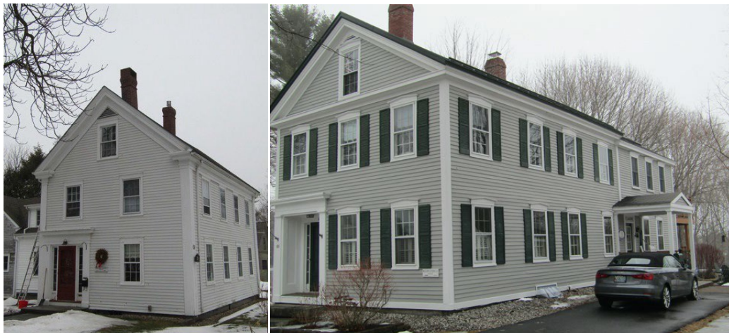
Above left, Daniel M. Stubbs House, 50 Pleasant Street. Gooding family members owned 68 Pleasant above right
