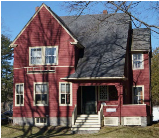
Captain Claudius Lawrence House, 111 West Elm Street. 151 West Elm Street.
