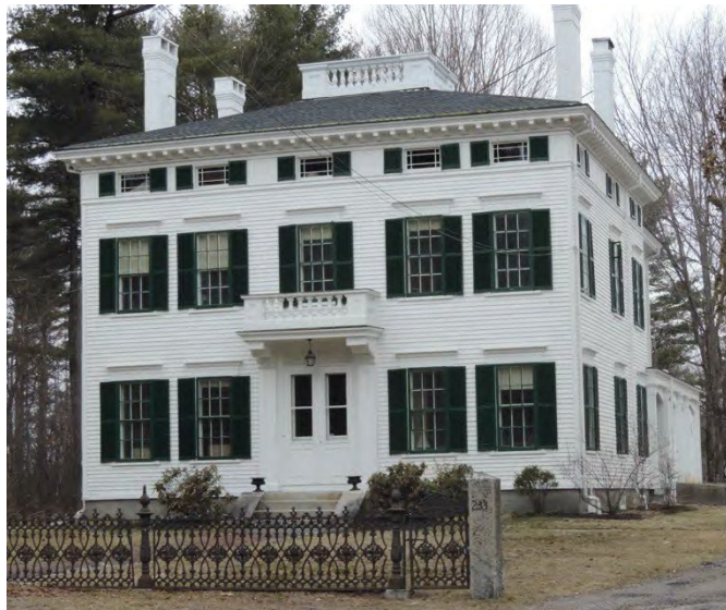
Captain Reuben Merrill House, 233 West Main Street.
