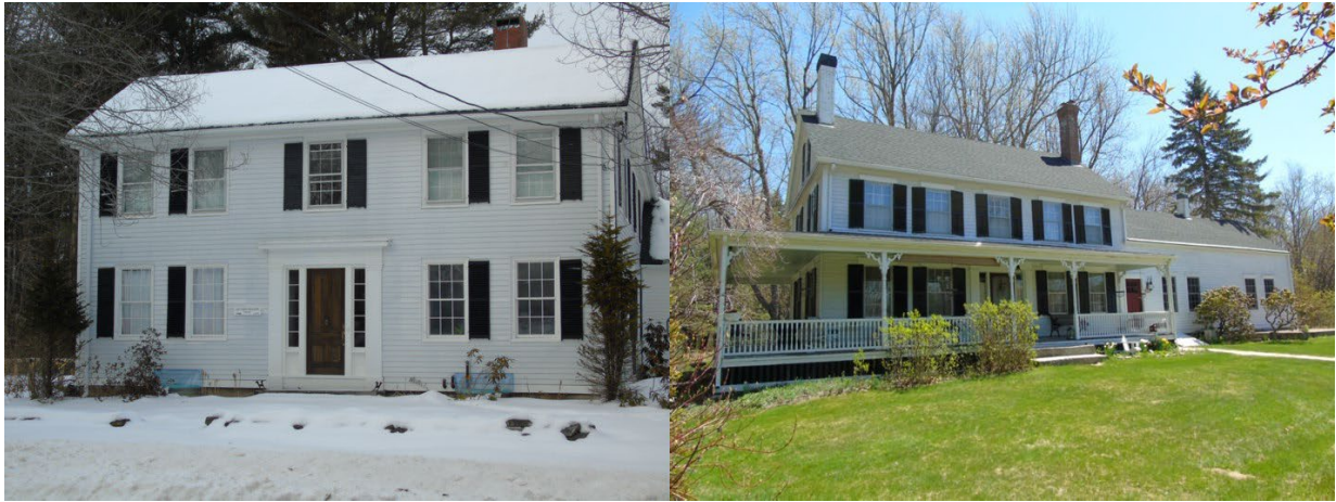
Captain Joseph Drinkwater House, 146 Gilman Road
