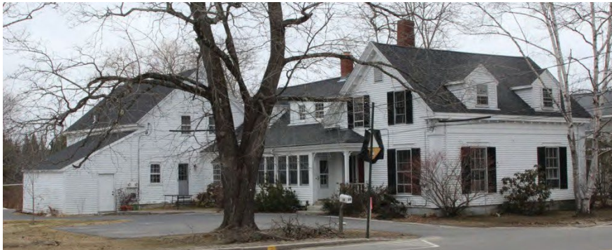
Nathaniel Gooch House & Barn, 30 East Elm Street.
