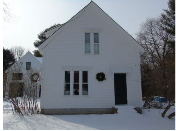
George A. Allen House, 119 Princes Point Road
