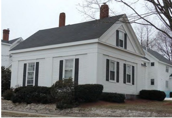
Coastal Manor Nursing Home, 20 West Main Street.
