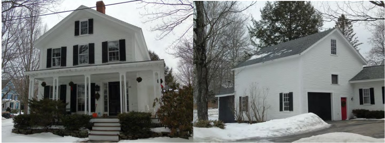
Edward H. Smith House & Barn, 65 Center Street.
