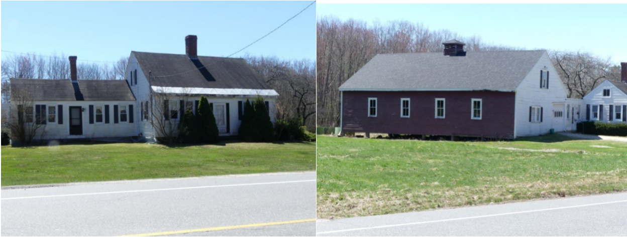
Allen Drinkwater House and Barn, 299 Gilman Road.
