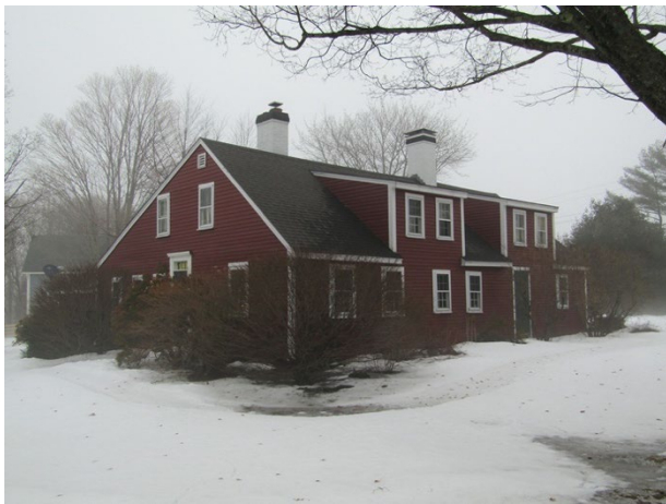
112 Pleasant Street, one of the earliest houses in Yarmouth, and its barn
