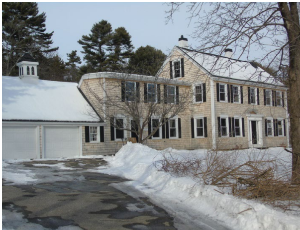
John Young House, 24 Gilman Road
