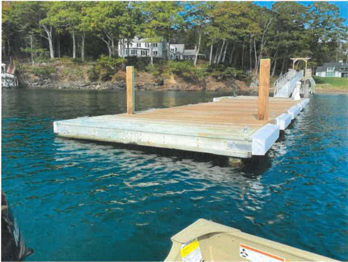
Photograph One: View of the Benson floats as currently installed. Please note the discoloration on the end float indicative of constant wave action overtopping the float.
