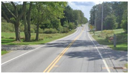
North Rd before hill up to train tracks, looking south
