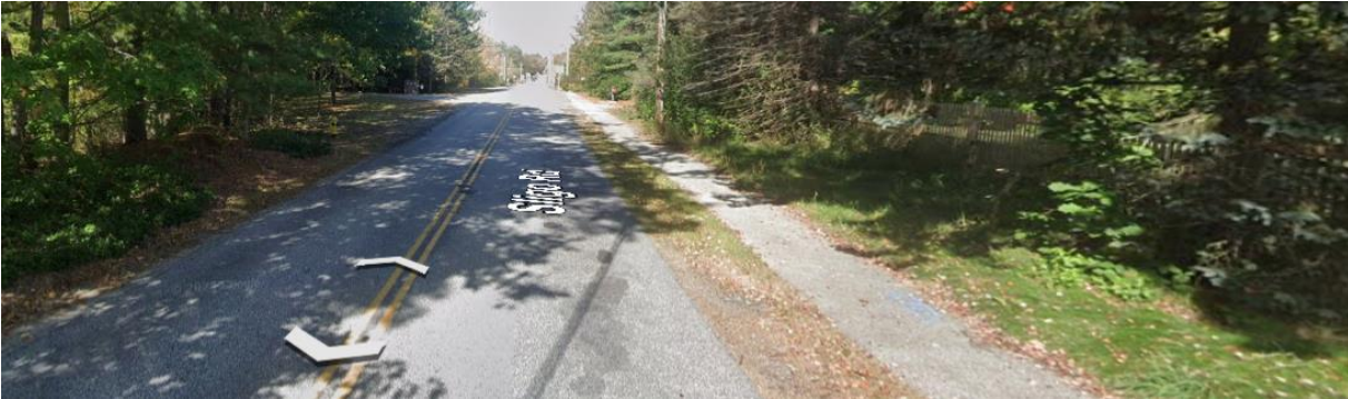
Sligo Rd looking west towards the railroad tracks
