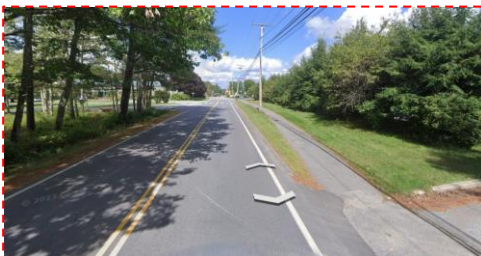
East Elm St at Leighton Rd, looking North
