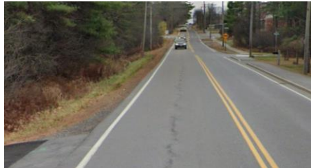
North Rd at Melissa Dr from the pump station, looking south
