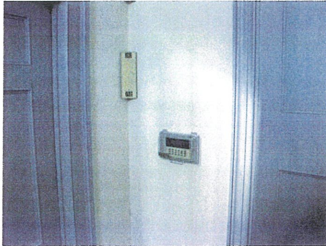
Figure 24 Narthex security console and sensor
