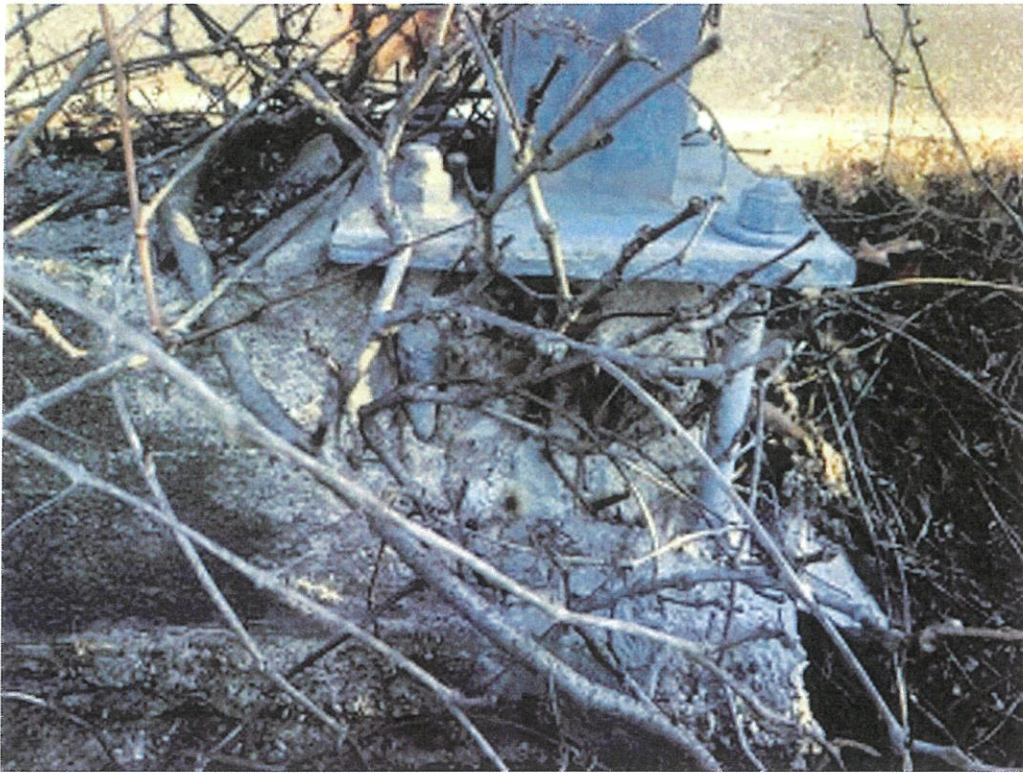
#338 Hodson Bridge: Note spalling at guardrail connections
