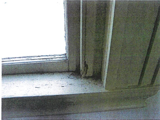
Figure 20 Sanctuary window interior showing paint wear from condensation
