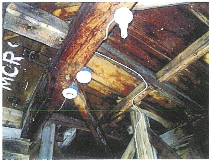
Figure 33 Attic electrical and fire sensors
