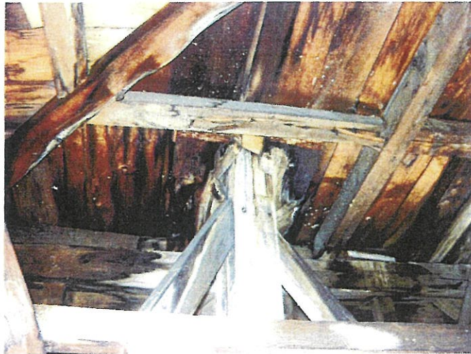
Figure 34 Steeple support penetration
