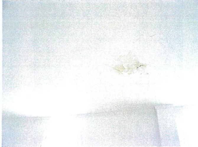
Figure 30 Water stain on second floor. Inactive leak
