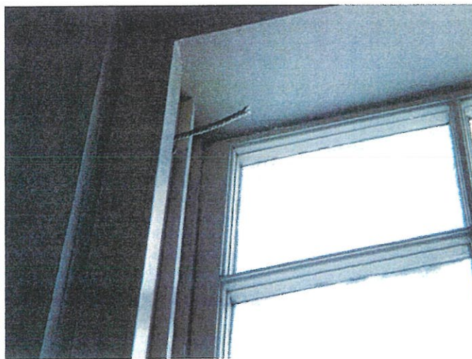
Figure 11 Broken rope on sanctuary triple hung window
