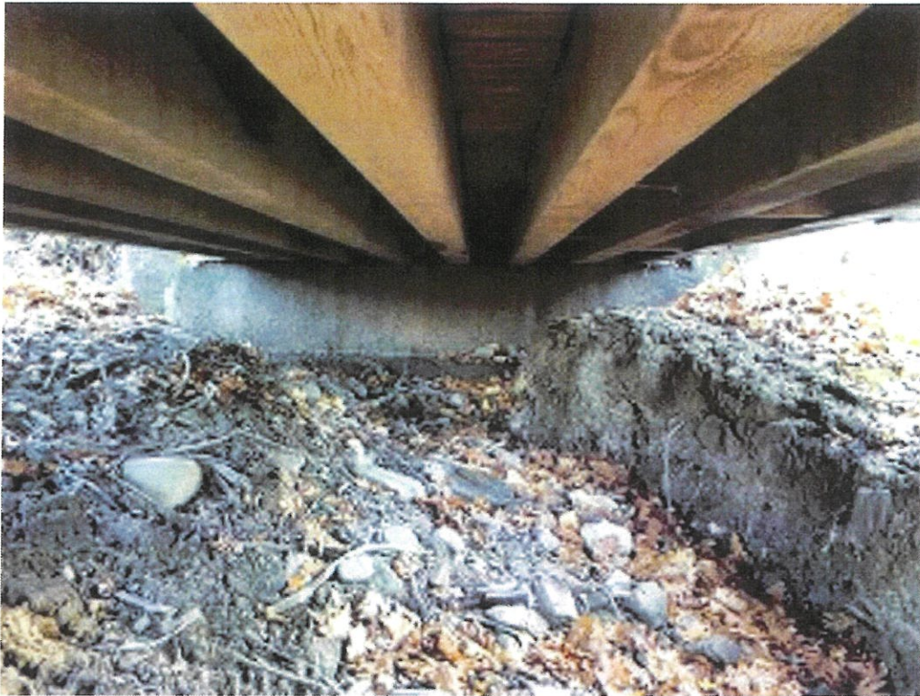
Dahlgren Bridge: View of erosion adjacent to the southerly abutment.
