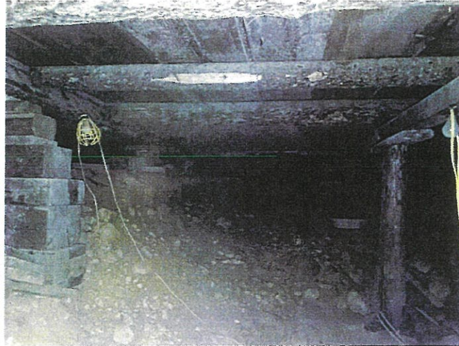
Figure 8 Crawlspace showing support piers and joists
