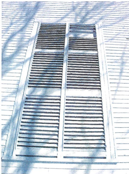
Figure 5 Louvered panel showing damage
