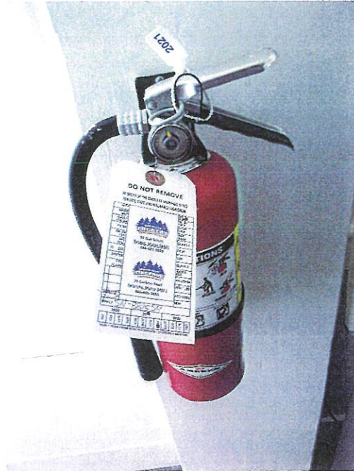
Figure 36 Fire extinguisher in need of inspection
