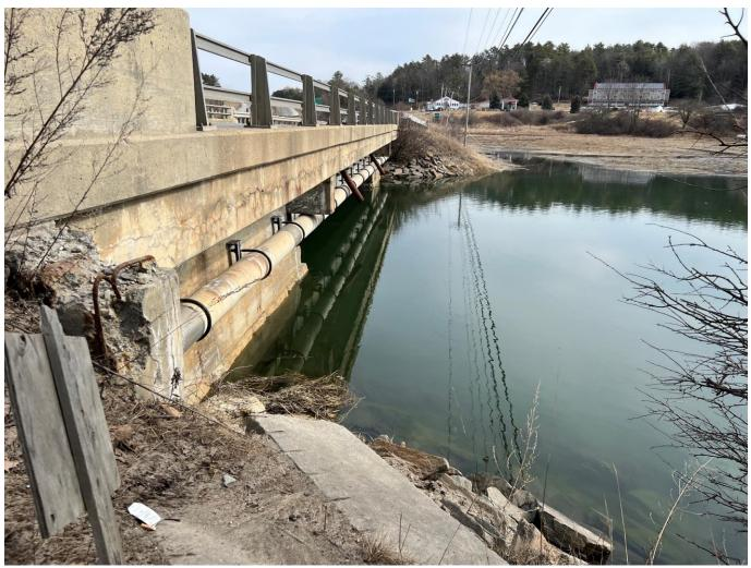
Photo 2 View of Cousins River and existing water main hung from US Route 1 bridge looking northeast toward Freeport (March 2023)
