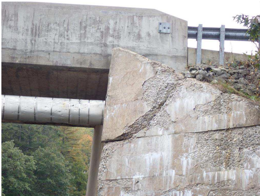
View of southwest wingwall: Note large crack.
