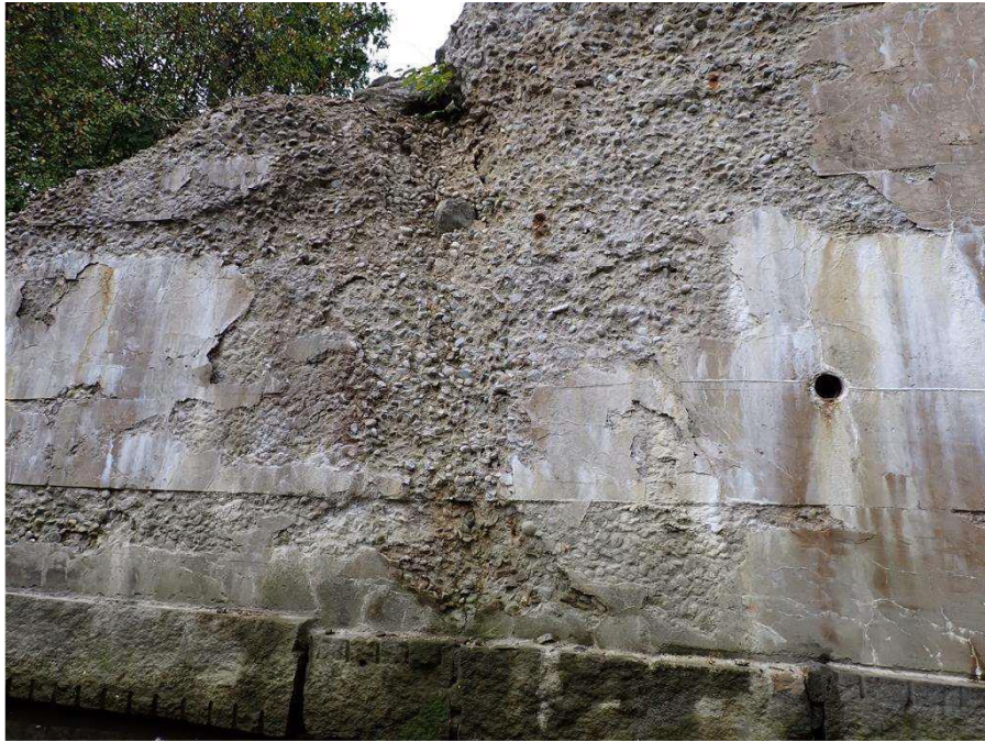
View of southeast wingwall: Note section loss
