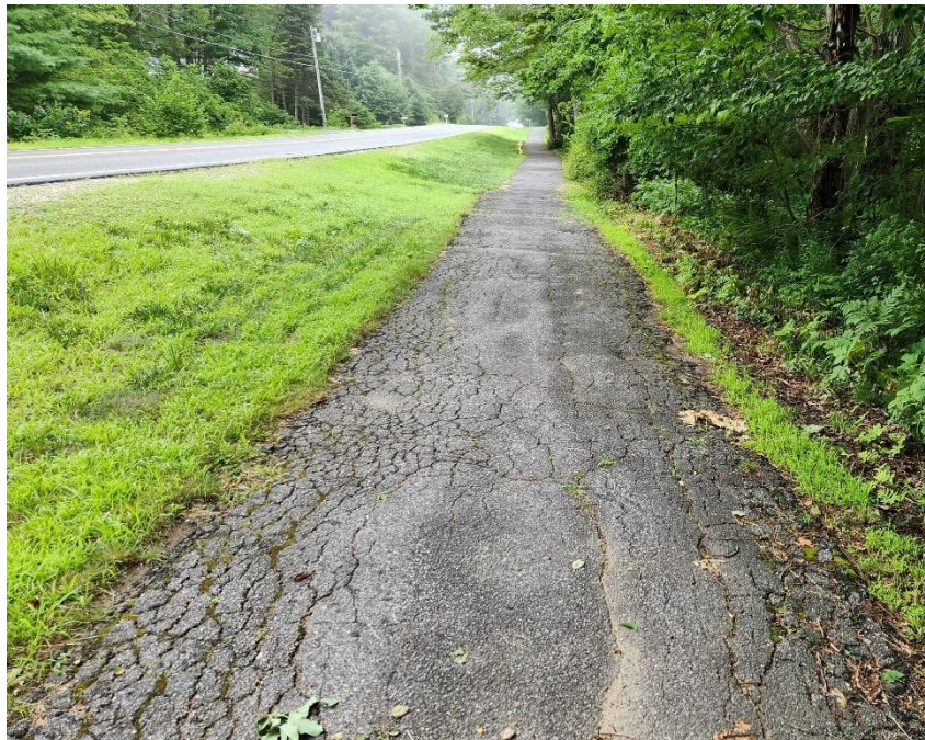
Note alligator cracking and uneven surface.
