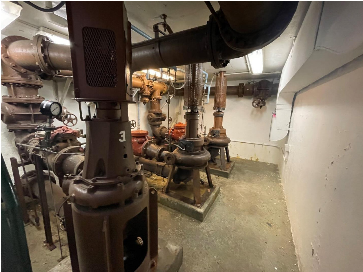
View of pump gallery in lowest elevation of the Harbor Pump Station
