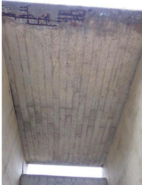
View of deck bottom: note exposed and corroded reinforcing steel.
