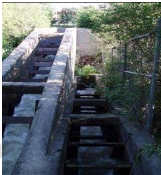
Figure 11: Denil-type Fish Ladder Near the East Elm Street Dam
