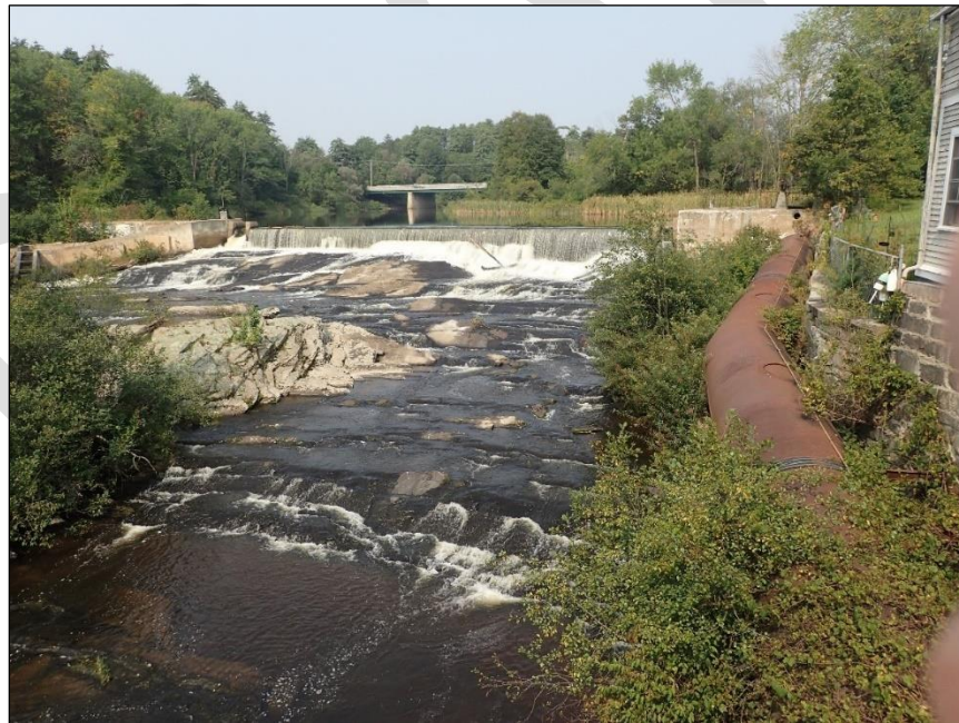
Figure 3: Bridge Street Dam & Fish Passage, Royal River, Yarmouth, Maine
