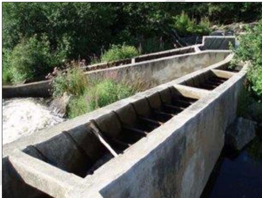
Figure 5: Denil-Type Fish Ladder at the Bridge Street Dam
