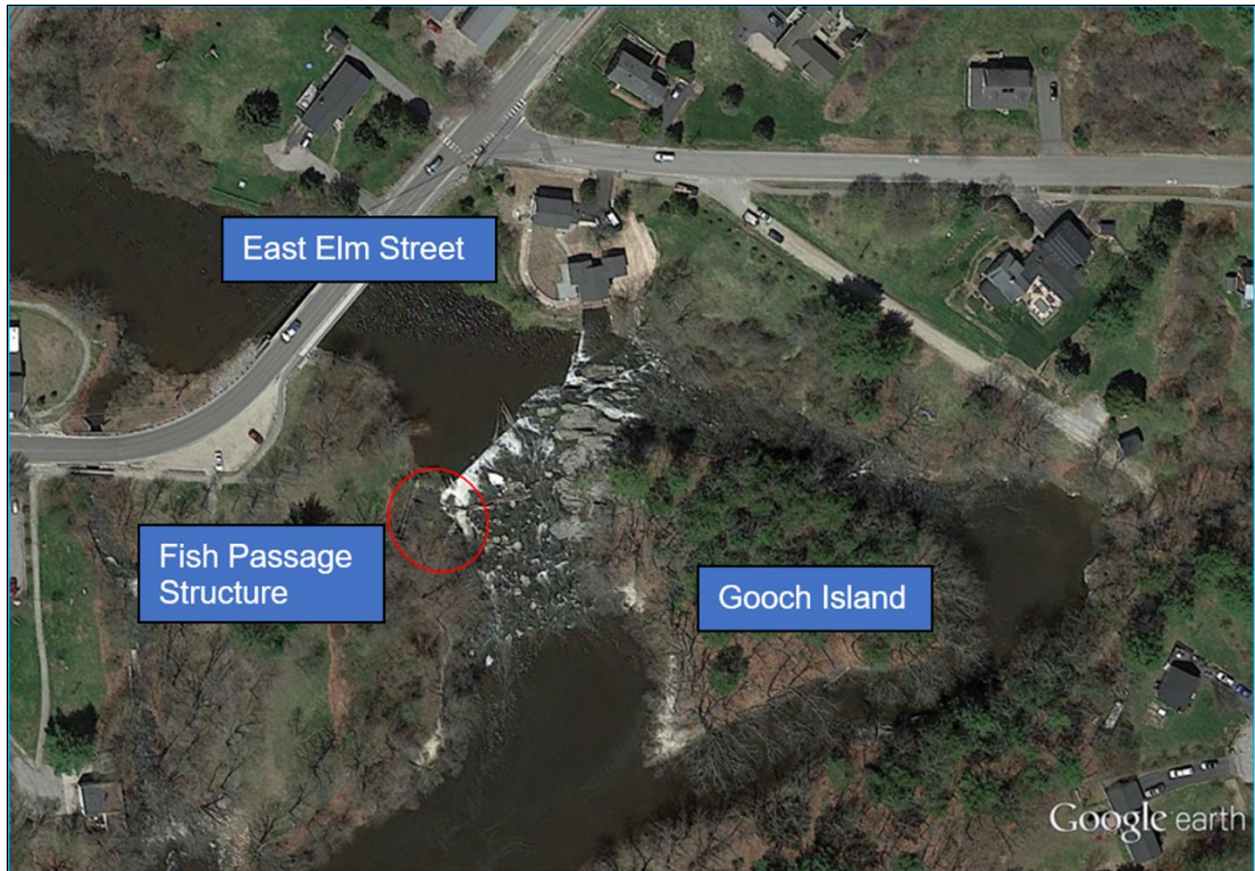
Figure 10: Aerial View of the East Elm Street Dam
