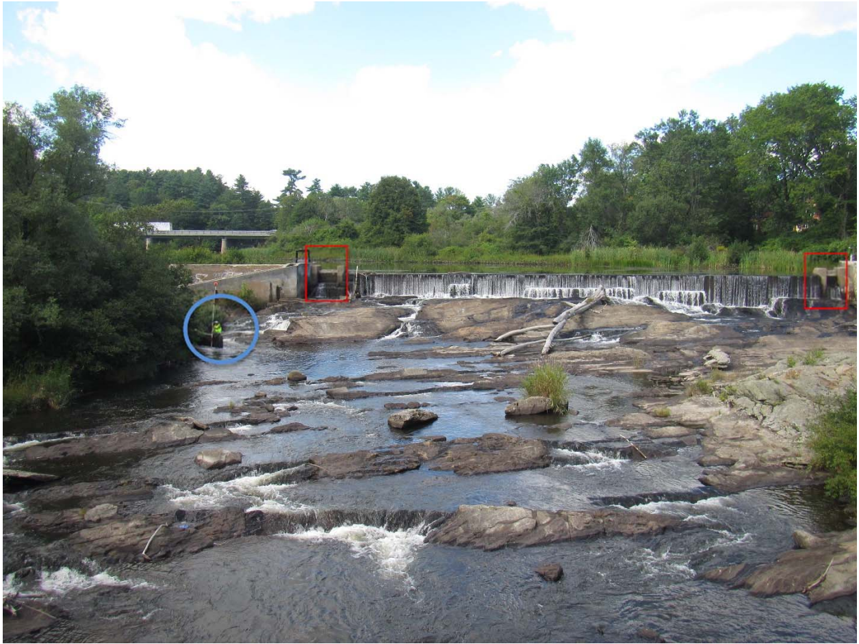
Figure 4: View looking upstream at Bridge Street Dam. Stop log weirs are indicated within the red squares and fishway entrance is indicated with a blue circle. Note surveyor for size. Flow direction is toward viewer.
