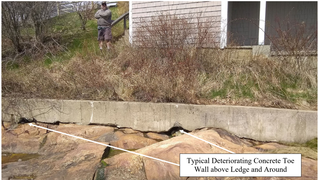
Looking north at a section of the deteriorating concrete toe wall to the east of the granite block seawall. Low Tide 1:27pm [Photo Time – Date: 11:00am – 4/16/20; Ebb Tide]
