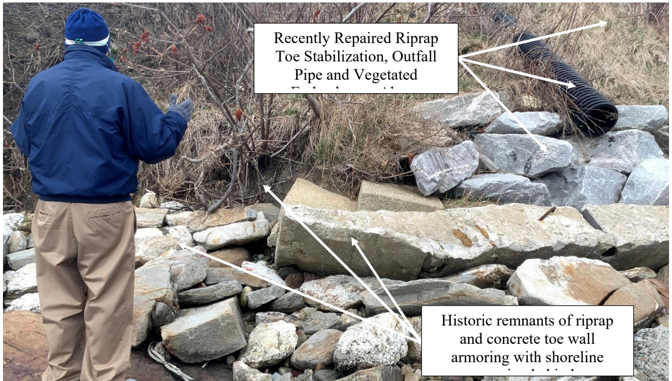
Looking north at a portion of riprap toe armored shoreline. Area to the right with the outfall pipe was part of the 2014 slope failure repair. Low Tide 1:27pm [Photo Time – Date: 11:00am – 4/16/20; Ebb Tide]
