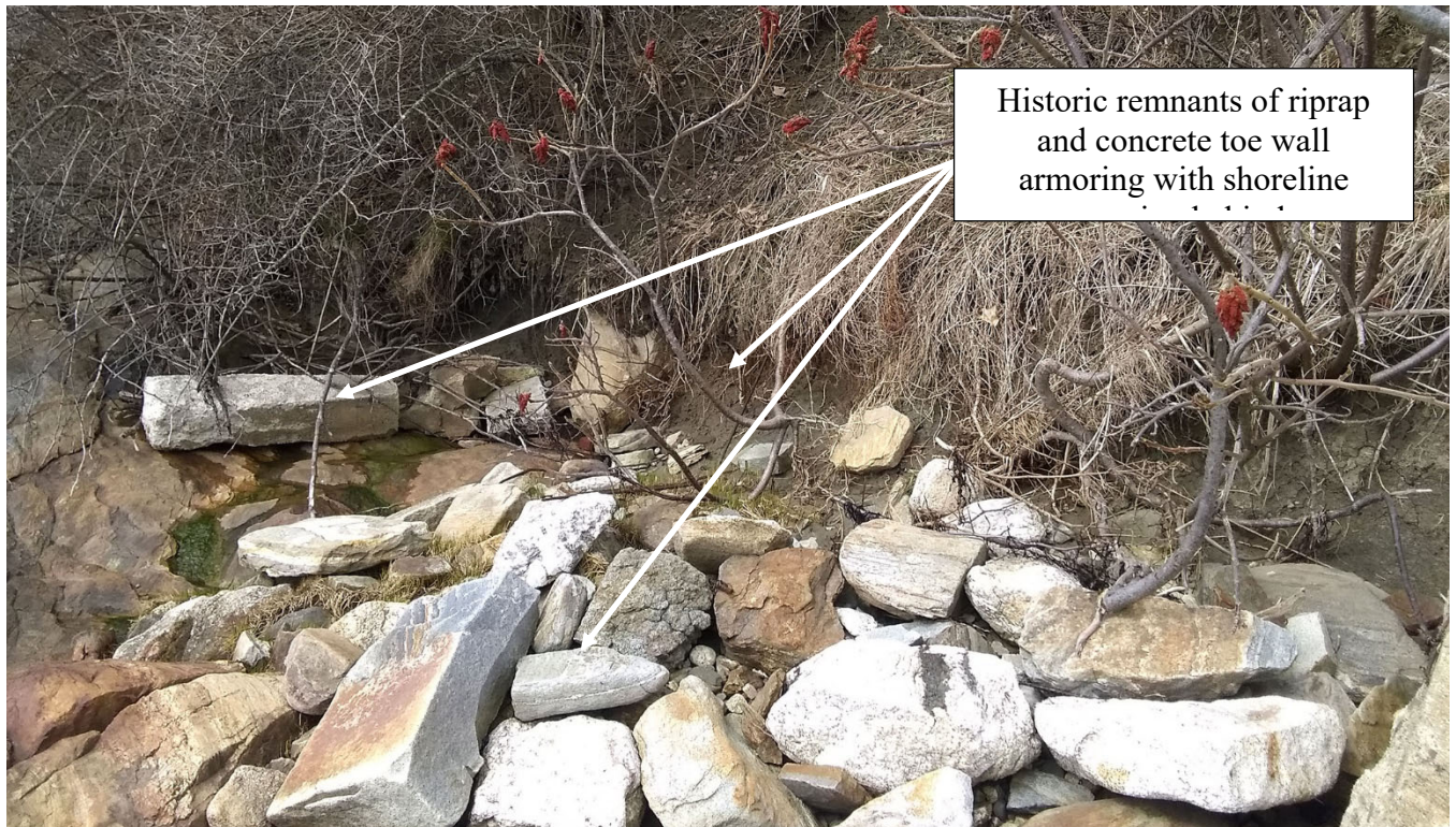
Looking northwest next to the slope failure repair where displaced riprap and deteriorated concrete toe wall conditions are occurring. Low Tide 1:27pm [Photo Time – Date: 11:00am – 4/16/20; Ebb Tide]
