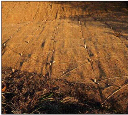
Figure 2 – Detail view: recommended buffer strip stabilization methods for 30 ft.-wide area landward of reconstructed revetment.
