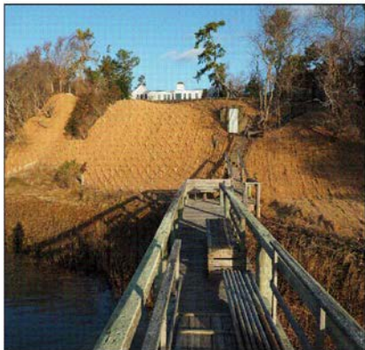
Figure 1 – Recommended 100% biodegradable stabilization methods for 30 ft-wide area landward of reconstructed revetment.
