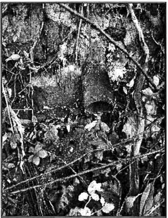
Existing Outflow Pipe - Mitigate Erosion With Fabric & Onsite Rock Material
