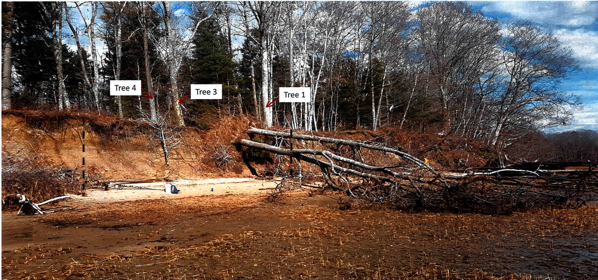
View northeast of eroding bluff, scarp, and fallen trees along the Lane's Island, Yarmouth demonstration treatment site. Approximate project boundaries shown with black dashed line. Trees labeled have been identified for potential removal during regrading and include: 1 (Oak, 26.4" DBH); 2 (Oak, 3.0" DBH); 3 (Oak, 13.4" DBH); 4 (Oak, 7.4" DBH). Tree 2 not visible in image. Image by P.A. Slovinsky, 12/3/2018.
