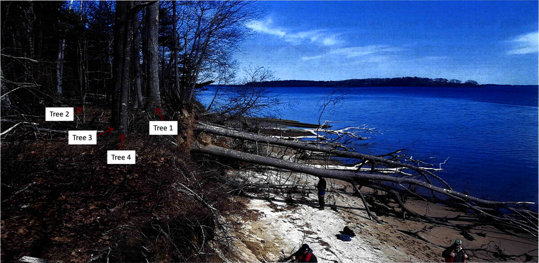
View east of eroding bluff, scarp, and fallen trees along the Lane's Island, Yarmouth demonstration treatment site. Trees labeled have been identified for potential removal during regrading and include: 1 (Oak, 26.4" DBH); 2 (Oak, 3.0" DBH); 3 (Oak, 13.4" DBH); 4 (Oak, 7.4" DBH). Image by P.A. Slovinsky, 4/11/2019.
