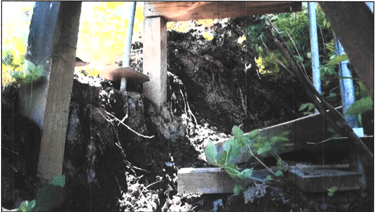
Photograph Four. View of erosion that is occurring along shoreline, specifically by existing stairs. Photographer: Lisa Vickers, Atlantic Environmental, LLC Date: June 19, 2018.
