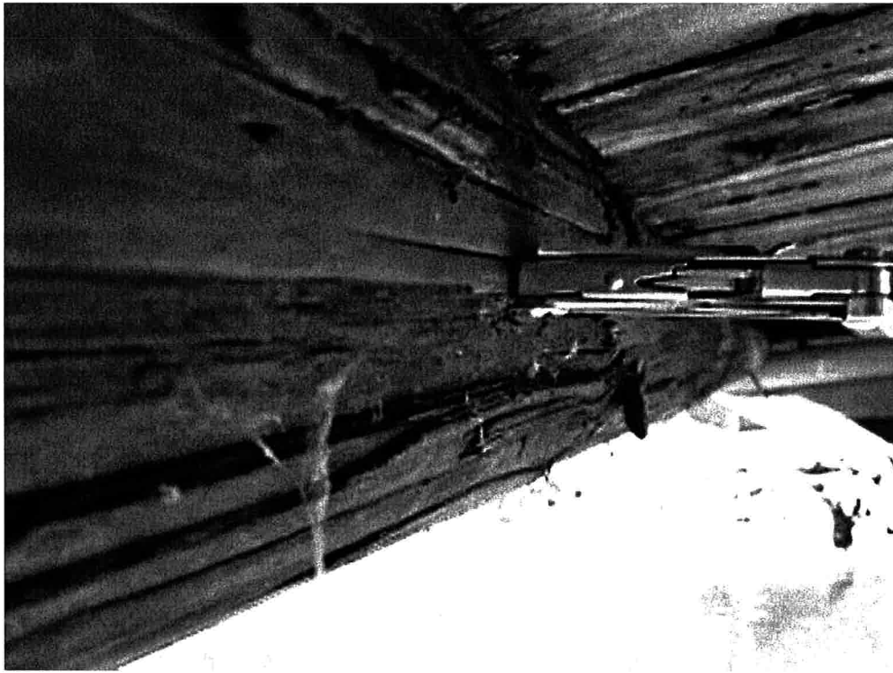
PB-4 Bear South Bridge Picture of downstream utility pole main structural member showing signs of significant deterioration and full probe insertion.
