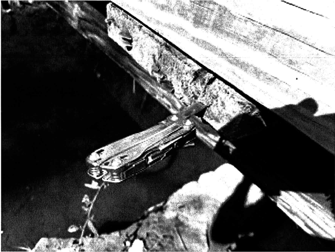
PB-4 Bear South Bridge: View of transverse member decay.
