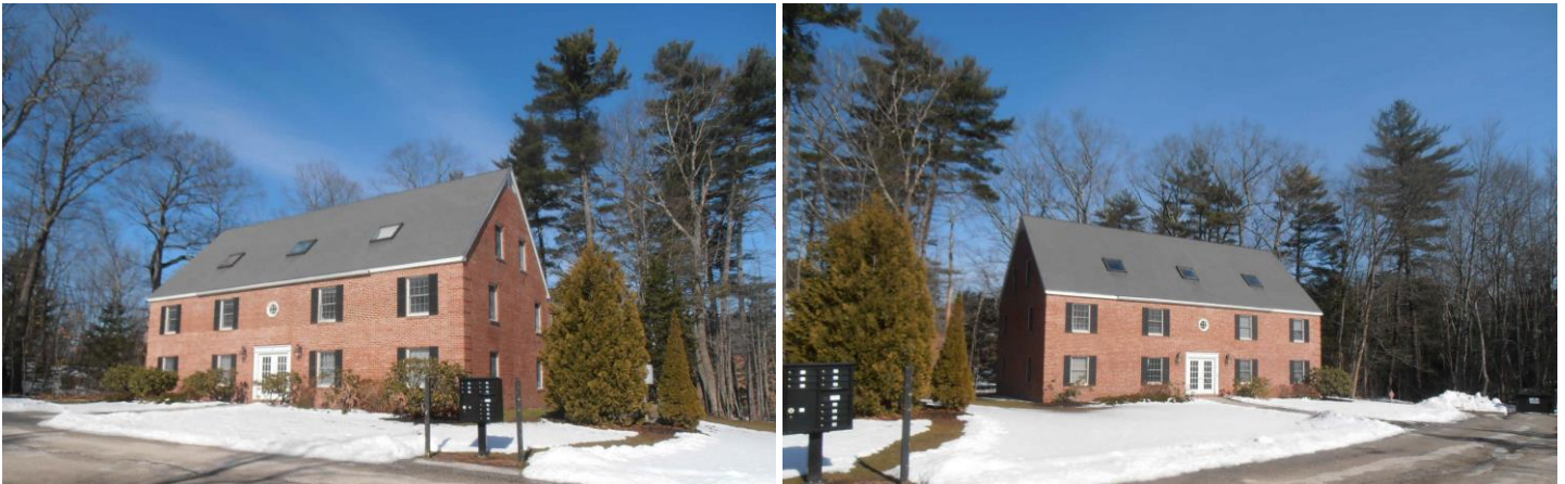
Existing Structures on the site; from the Assessor's Database
