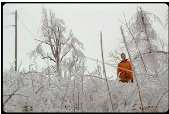
Figure 1 Frozen Power Lines - Ice Storm, Quebec, Canada 1999
