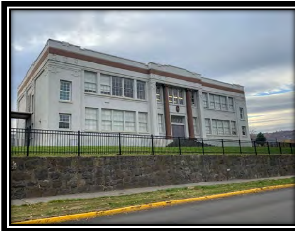
CWE Rod Iron Fencing Along 14th Street
