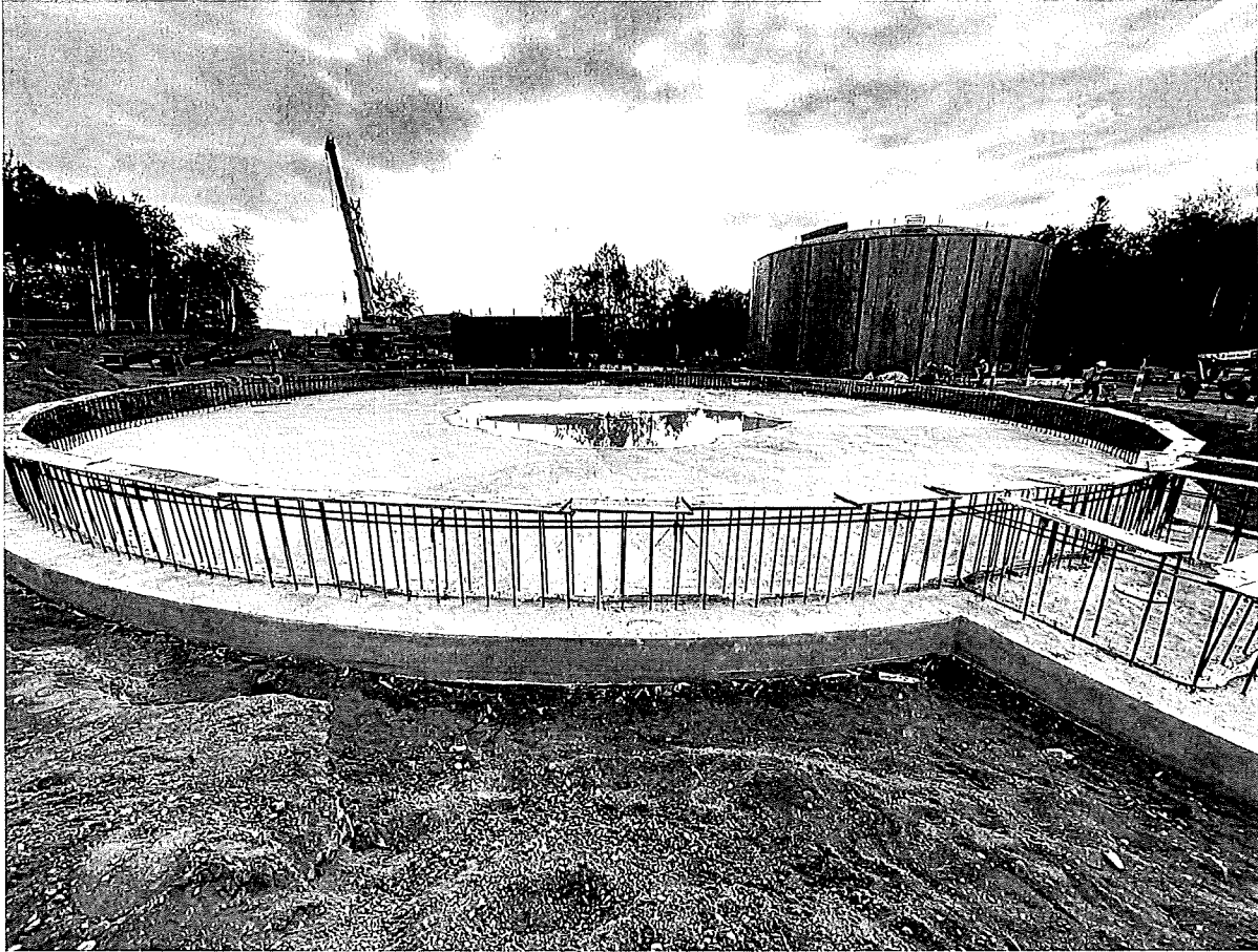
Clarifier #1 Base Slab Concrete
