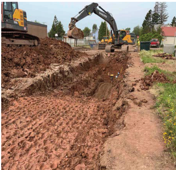
5 th Avenue Water Main Installation
