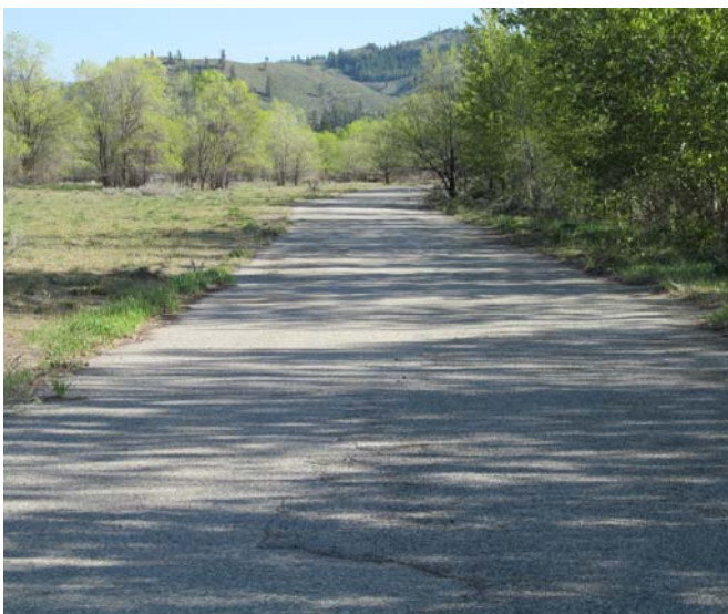
Old roadbed along east side of Methow River is ideal for development of a Shared Use Path
