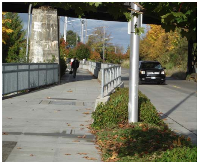
Guardrail separation where there are space constraints
