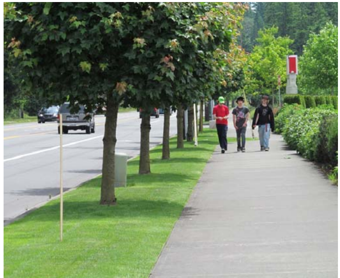
Planting strip and wide sidewalk
