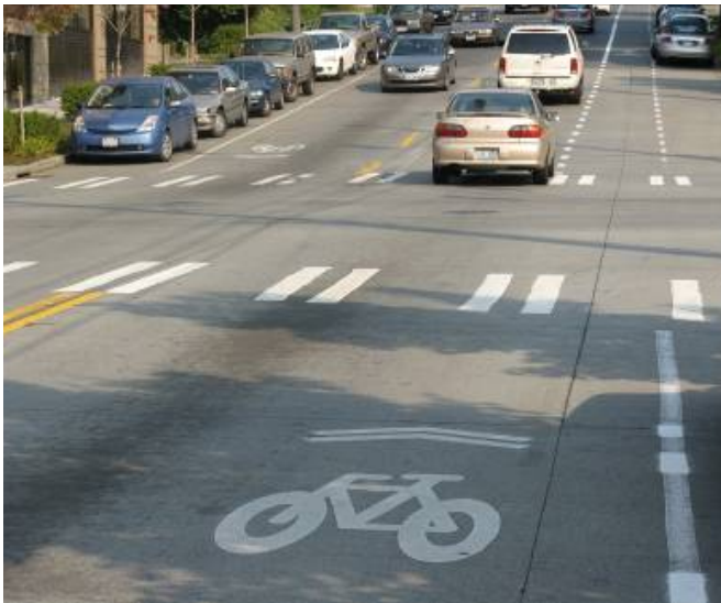
Marked Shared Lane transition to Bike Lane on an incline. Note transition is reversed in opposite lane
