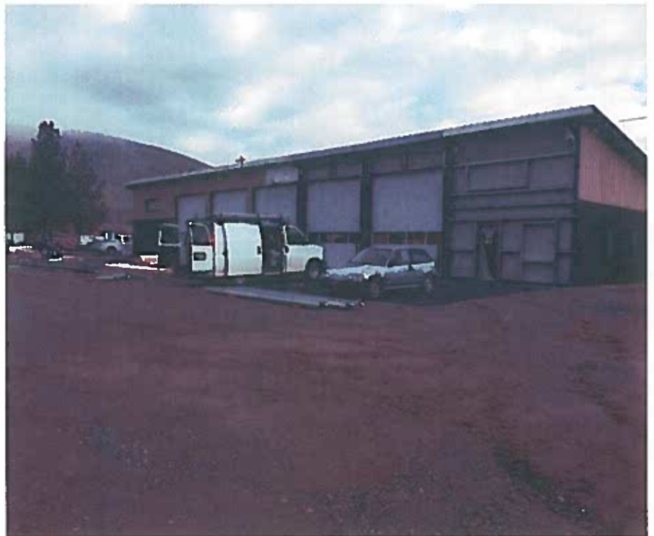
Public Works Shop (near completion)
