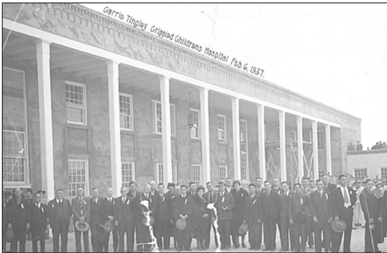
Carrie Tingley Hospital for Crippled Children Construction February 6, 1937
