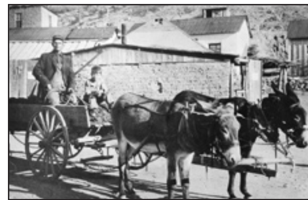
First Water System
