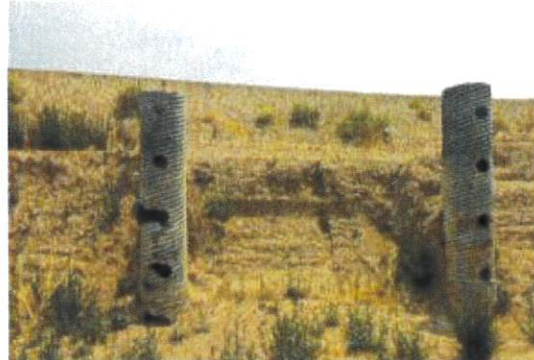
6. Condition of 2-24-inch standpipes. Left Standpipe is clogged. Looking south.
