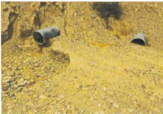
7. 2-24-inch standpipe outlet. Right outlet is clogged. Looking North.
