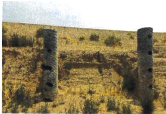
6. Condition of 2-24-inch standpipes. Left Standpipe is clogged. Looking south.
