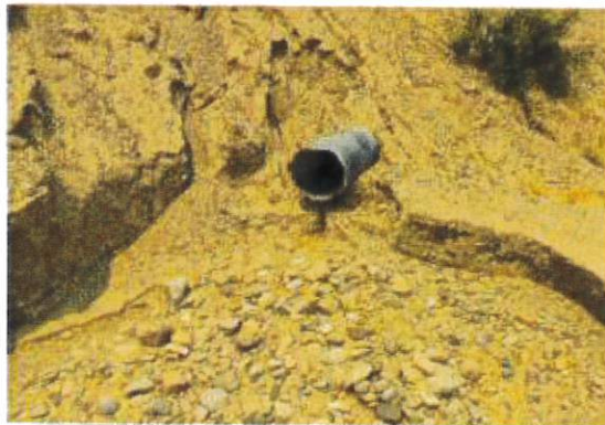
8. Close up of functioning standpipe outlet. Looking North
