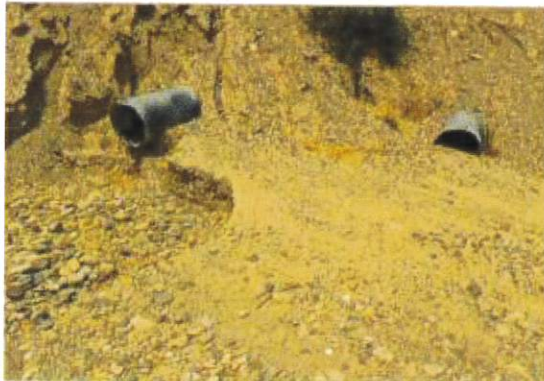
7. 2-24-inch standpipe outlets. Right outlet is clogged. Looking North
