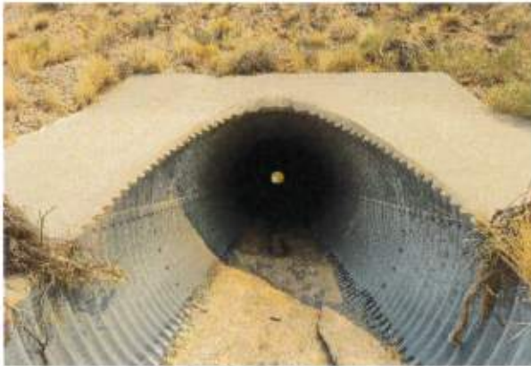
9. Headwall of 120-inch CMP Looking South Towards I-25
