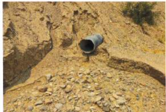
8: Close up of functioning standpipe outfall. Looking North
