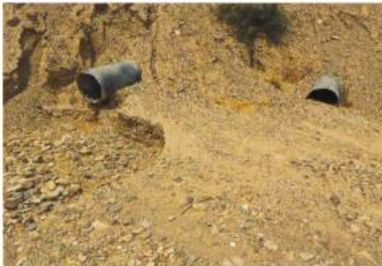
7: 2-24-inch standpipe outfall. Right outfall is clogged. Looking North
