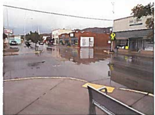
Ponding after a storm in Downtown.
