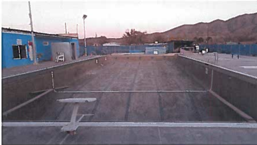
Old plaster completely removed New lane tiles installed
