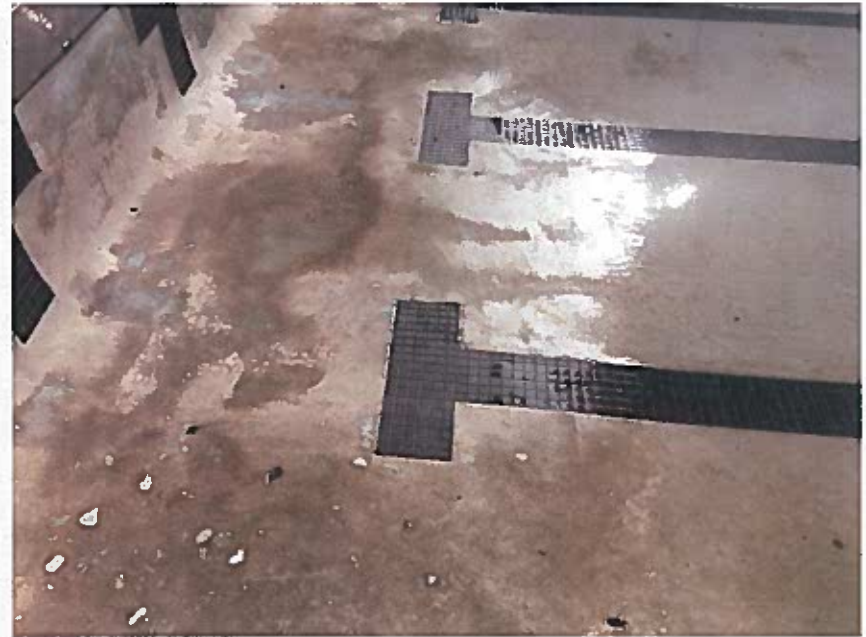
Close-up of chips in old plaster
