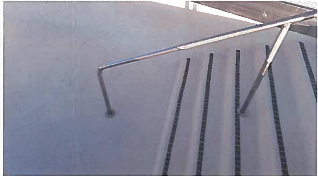
Handrail fixed – new anchors installed
