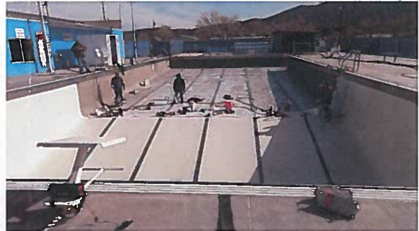
New plaster being installed
