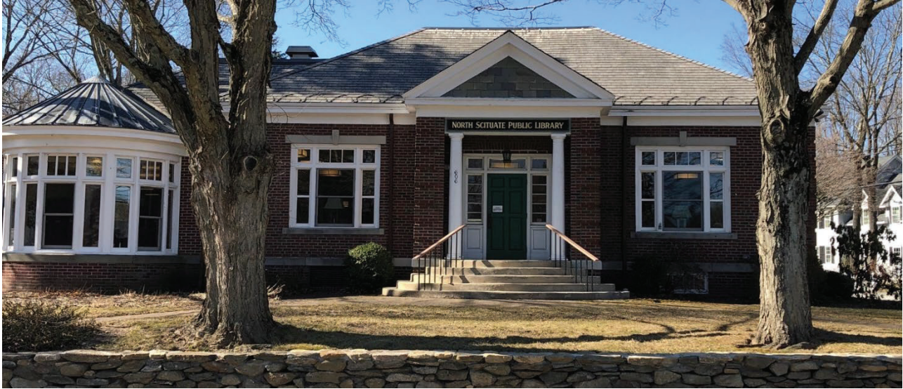
Figure 10-2. North Scituate Public Library
