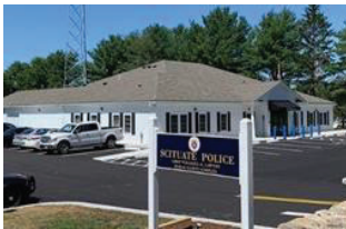
Figure 1. Scituate Police Station (Sugrue & Associates, Inc.)
