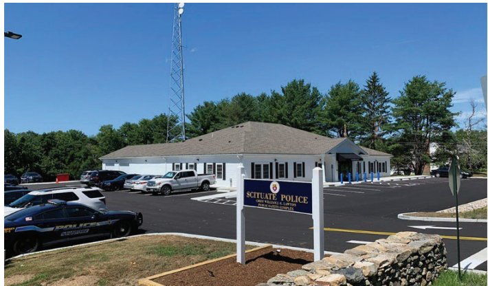
Figure 10-1. Scituate Police Station (Sugrue & Associates, Inc.)
