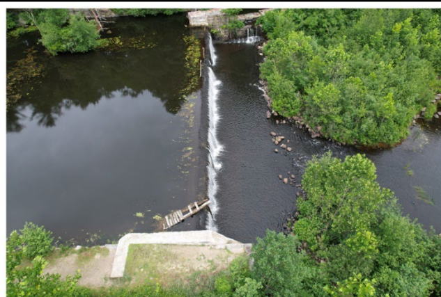
Hope Dam – showing debris
