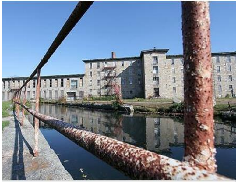
Figure 9-1. Hope Mill, 2016 Source: Valley Breeze (Retrieved on 7/1/21)
