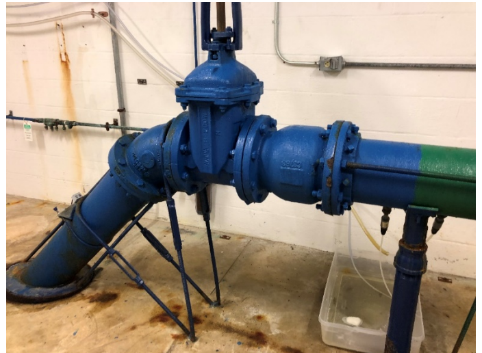
8-inch gate valve with backflow preventer.
