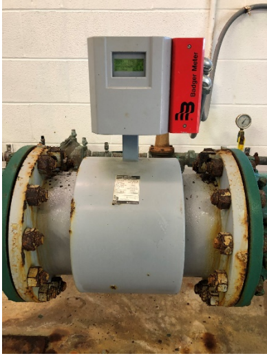
10" Magnetoflow Primo magnetic flow meter.
