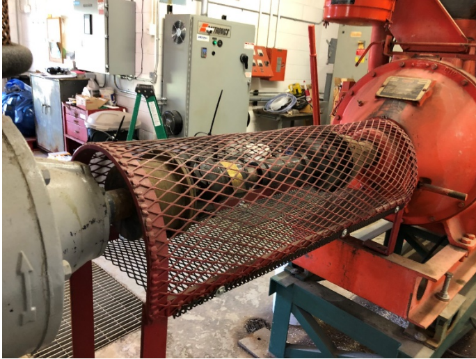
Connection between Well Pump 2 and the backup motor.
