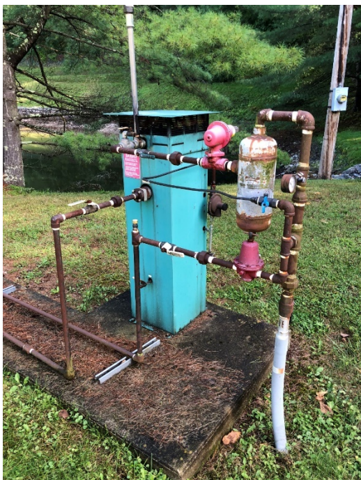
Gas piping for propane fuel delivery system.
