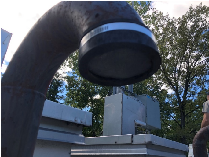
Tank vent is shown with wire screen guard.
