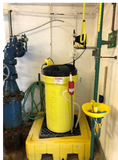
Treatment area inside well and pipe room for chlorine injection.
