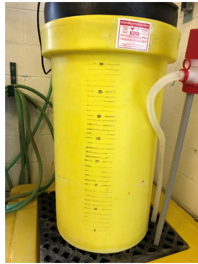
Chlorine 50-gallon storage tank.
