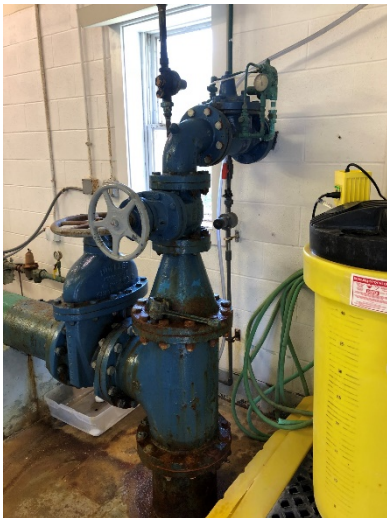
Blow-off assembly installed adjacent to the chemical injection area with 4" Cla-Val pressure reducing valve.
