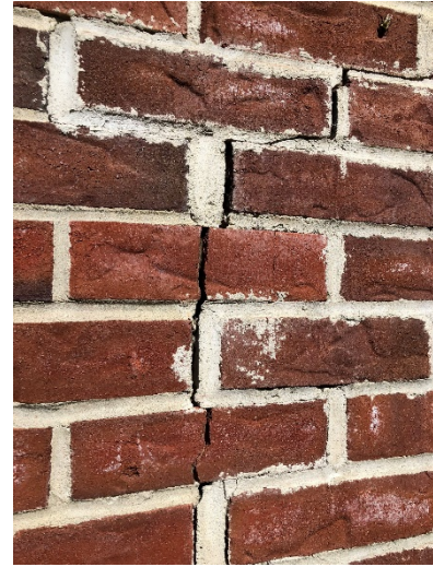
Cracking visible on the exterior of the building.
