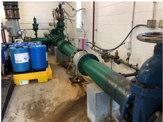
Chlorine storage area in pump room.
