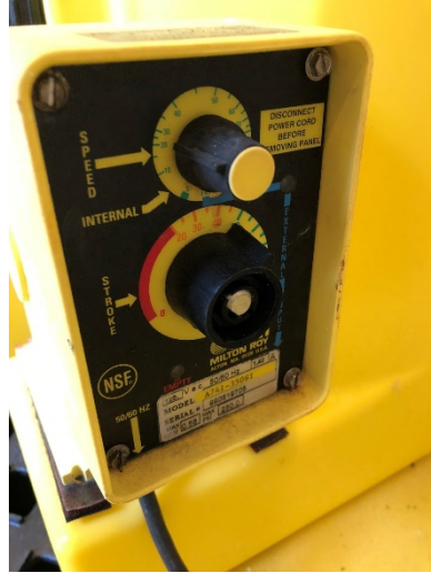
LMI hypochlorite feed pump
