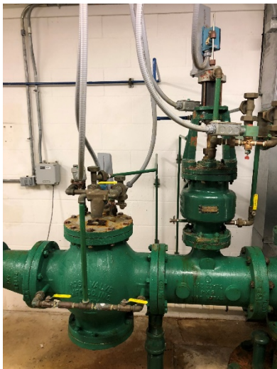
Pump control valve (left) and blow-off assembly (right).
