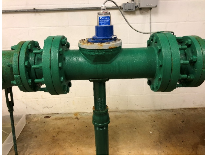
Sensus meter installed.
