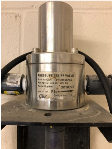
Pressure relief valve installed in treatment area.
