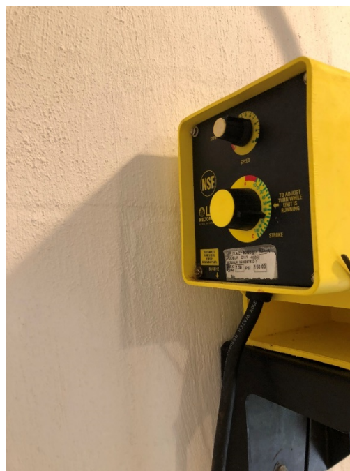
LMI fluoride feed pump.
