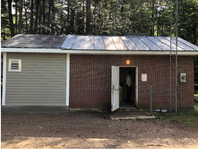
Front view of Well House 3 showing chemical room addition being constructed.
