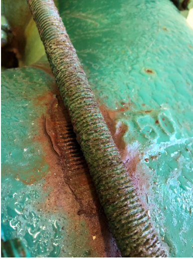
Wear on the fittings and pipe caused by the flexing of the threaded retainer rods.
