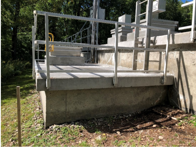
Access hatches and landing at the rear of the reservoir.
