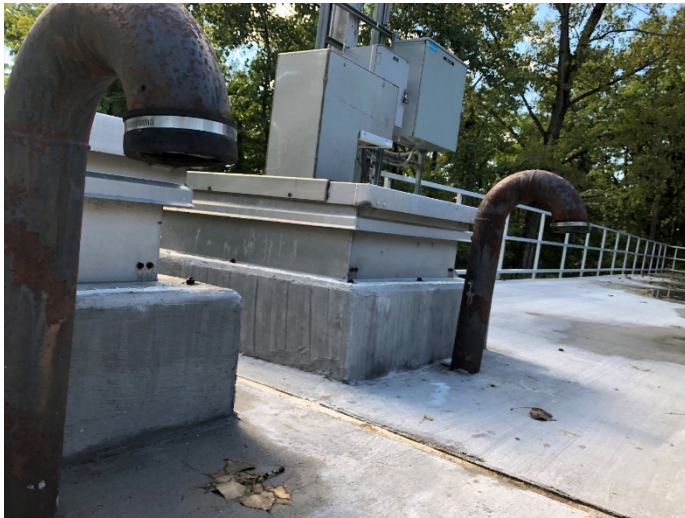
Access hatches for the reservoir showing vents.
