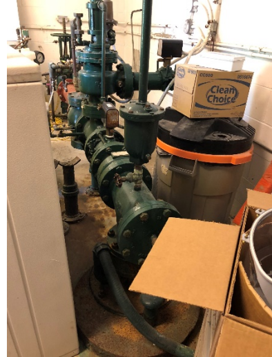
Well House 2 piping, showing the top of the submerged well in the foreground.
