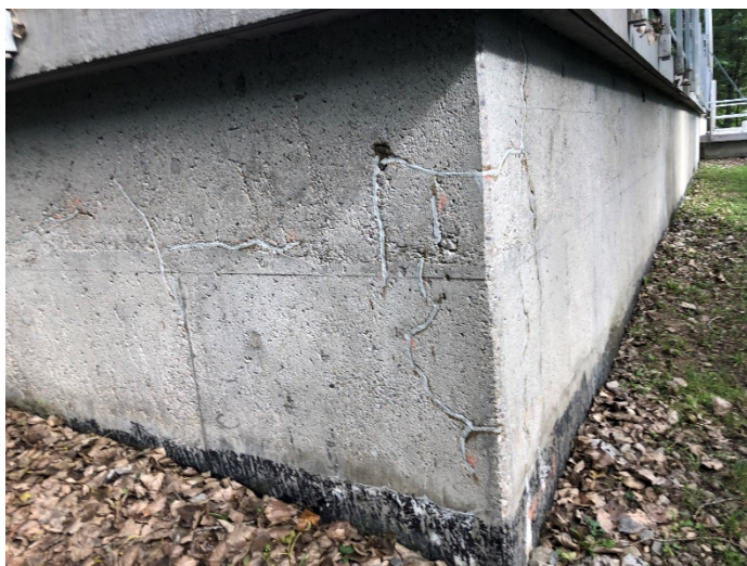
Repaired area on reservoir wall.
