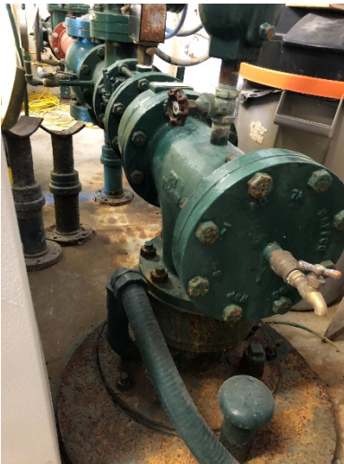
Close-up view of the cap on the submerged well.
