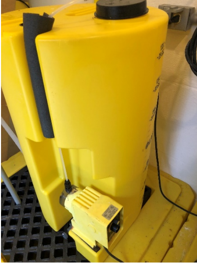
50-gallon hypochlorite tank with pump.
