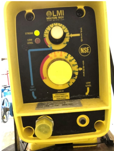
LMI chemical pump for chlorine injection.
