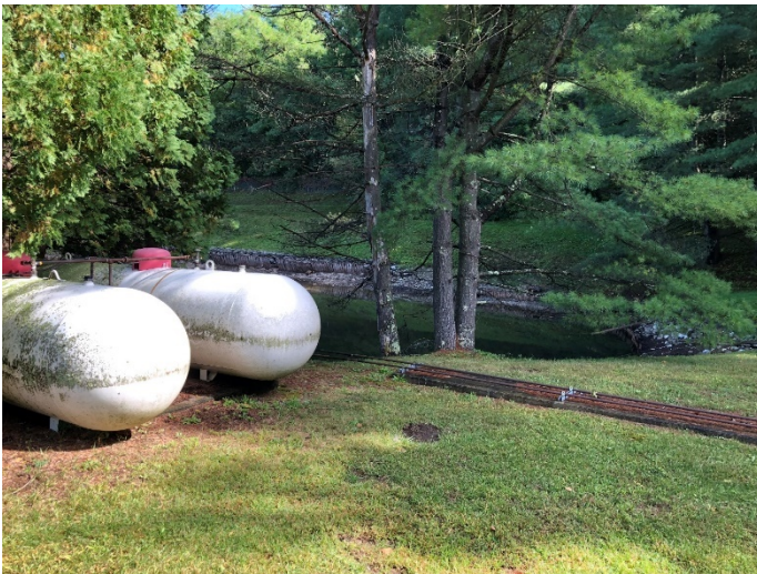
Propane tanks for backup power generation
