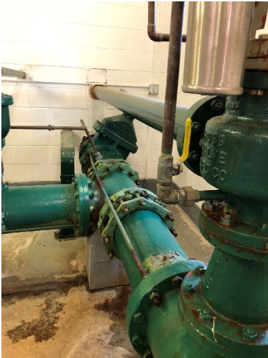
View of piping out of well pump. Threaded rods are installed for extra needed thrust protection.
