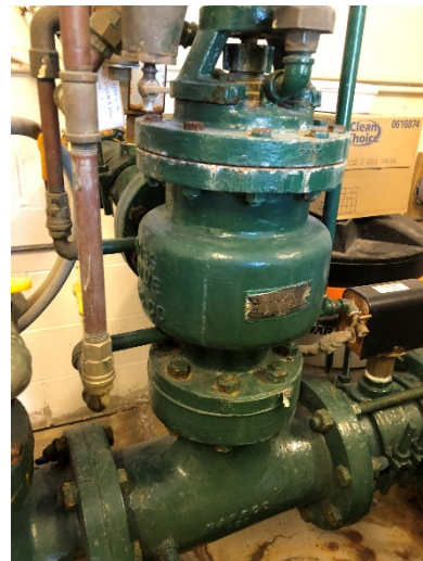
Backflow preventer valve is shown as part of the blow-off assembly.
