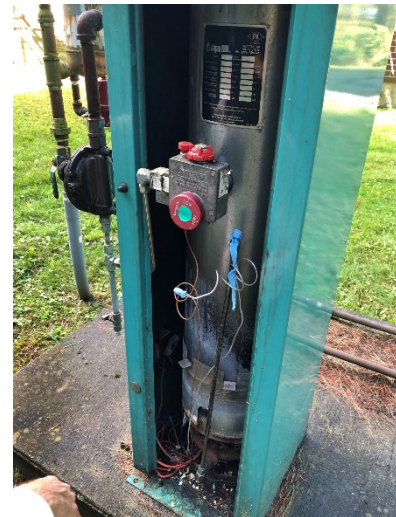
Phase changer for cold weather propane use.
