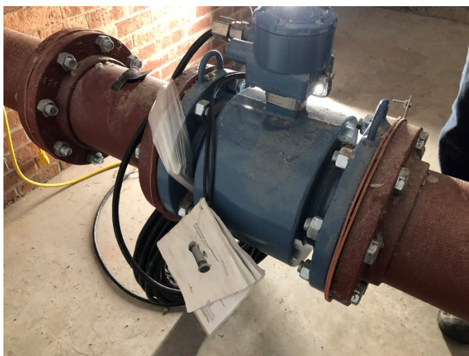
New Rosemount magnetic flow meter installed in the new treatment room.
