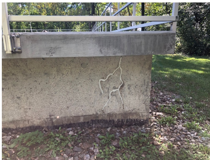
Repairs on reservoir wall.
