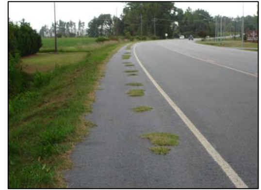
A bicycle lane in need of maintenance. Once bike facilities are constructed, they must be properly maintained.
