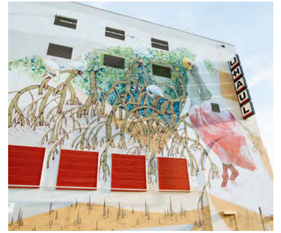
Image Credit: City of St. Petersburg
