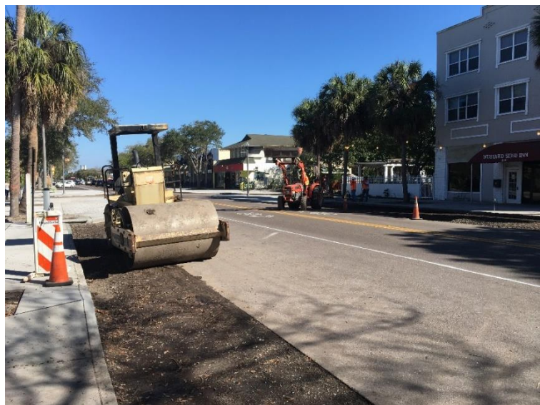
Example of Project Implementation
