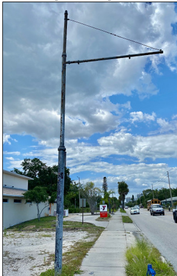
Original Steel Sign Pole
