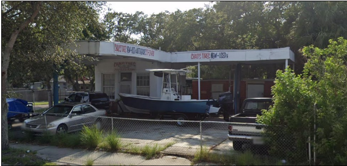
Figure 4: Google Streetview capture of the building from 2019, prior to rehabilitation.
