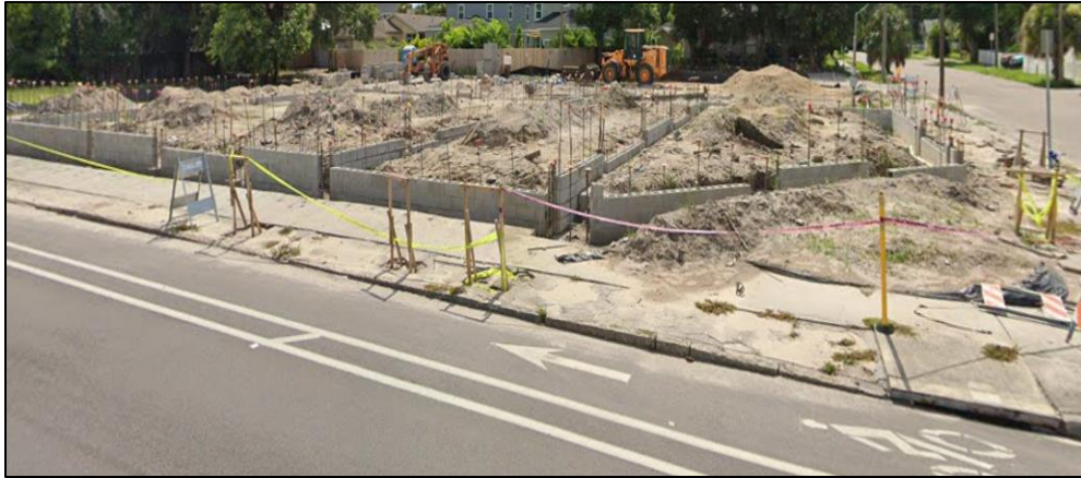
New foundation construction after demolition
