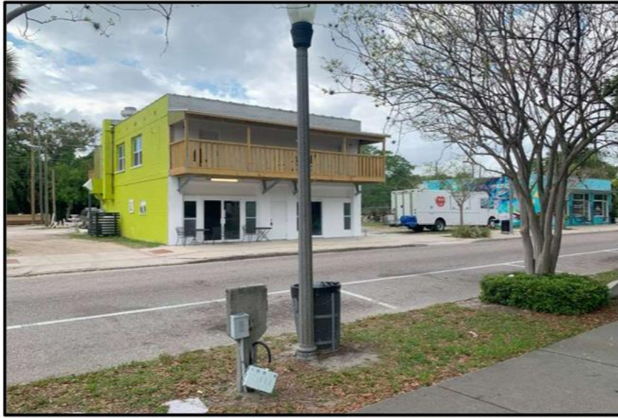
RECENTLY RENOVATED MADAM QUEEN BUILDING NORTH OF SUBJECT
