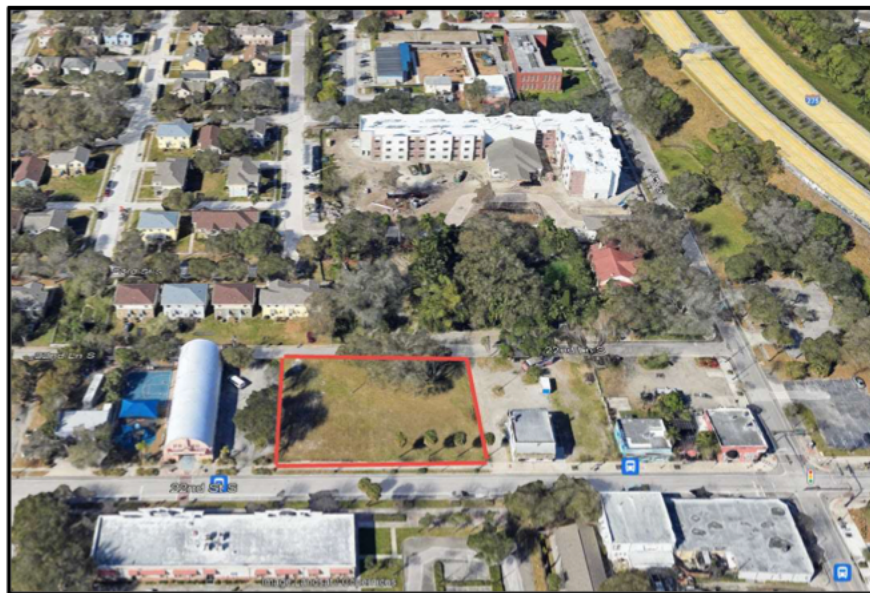
AERIAL VIEW FROM EAST
