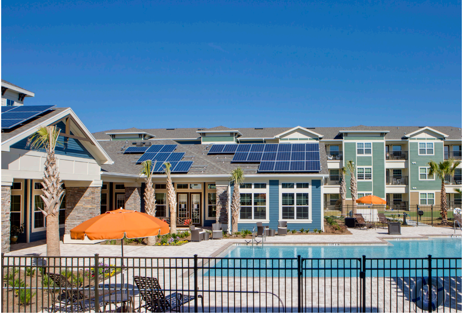
Forest Ridge Clubhouse - Solar Panels
